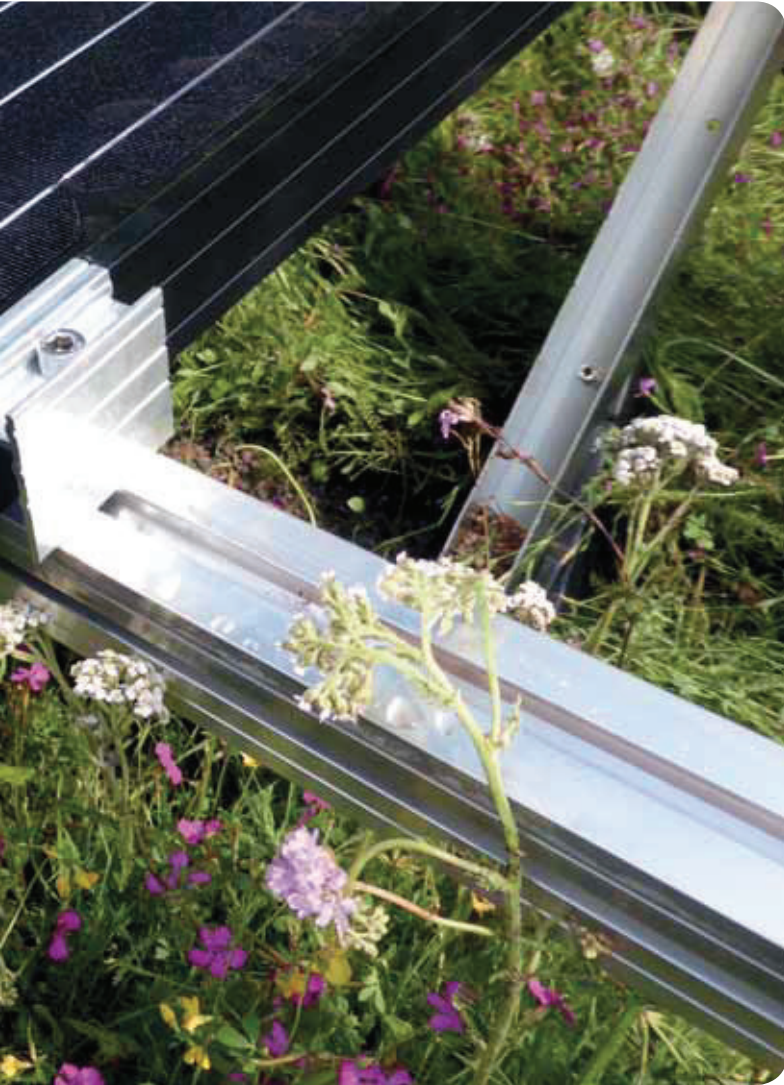
Mounted photovoltaic panel prior to the installation of the ballasting green roof and vegetation.
