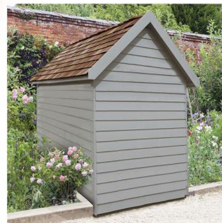
TYPICAL APPEARANCE OF SHED/ PLANT ROOM.
