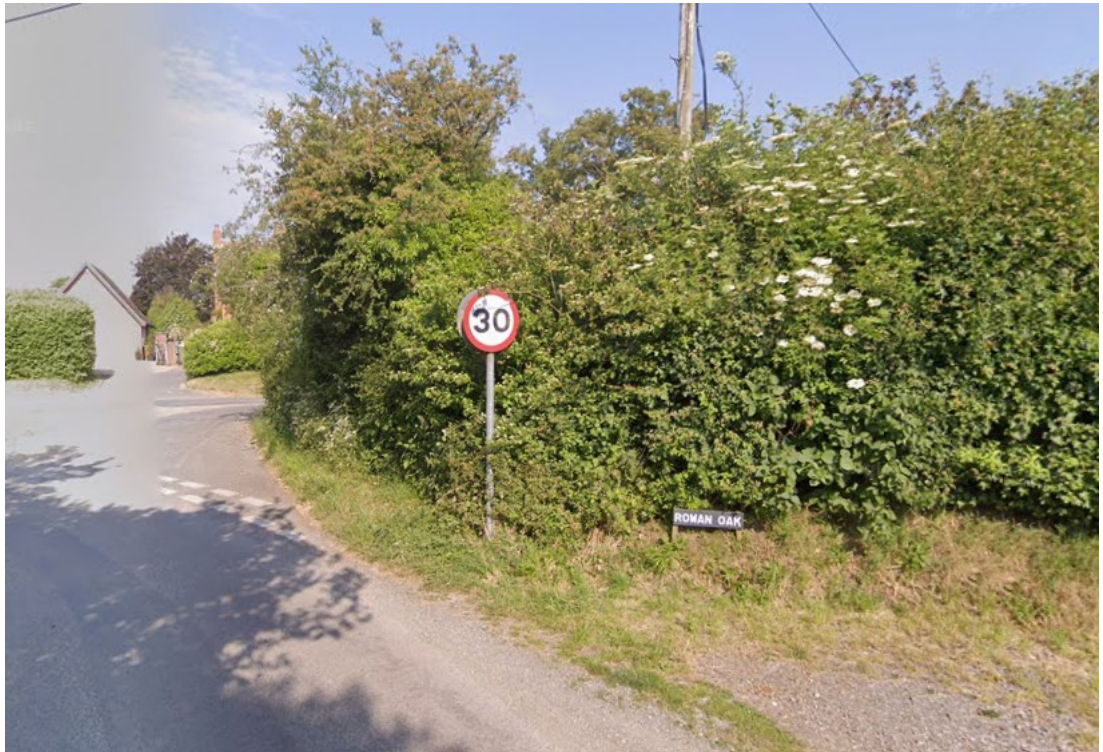
Figure 5: Highway verge ensuring good visibility
