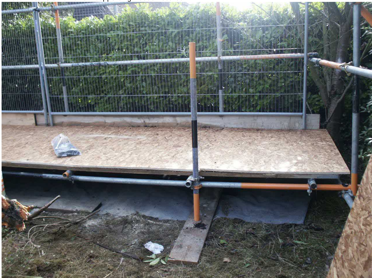
Photo 2 Scaffold framework supporting wooden boards
