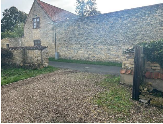
Access Point from Driveway
