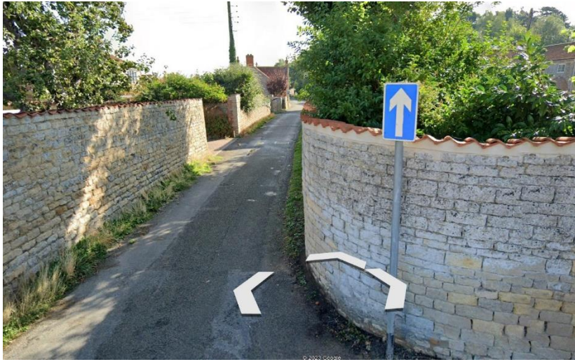
Back Lane facing entrance from Potterhanworth Road
