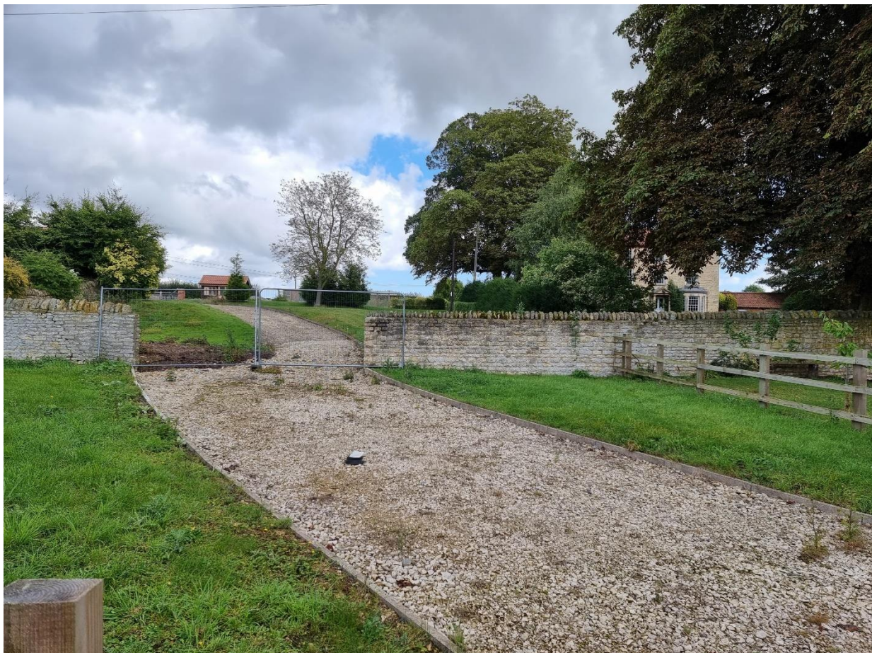
View from Far End looking east at existing stone wall and gate opening
