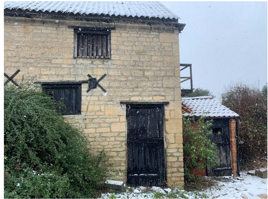
P13, right – original slatted breather vents (slide from side to side to control the flow of air). To the right, on the south elevation, a modern balcony floats above the brick outbuilding.
