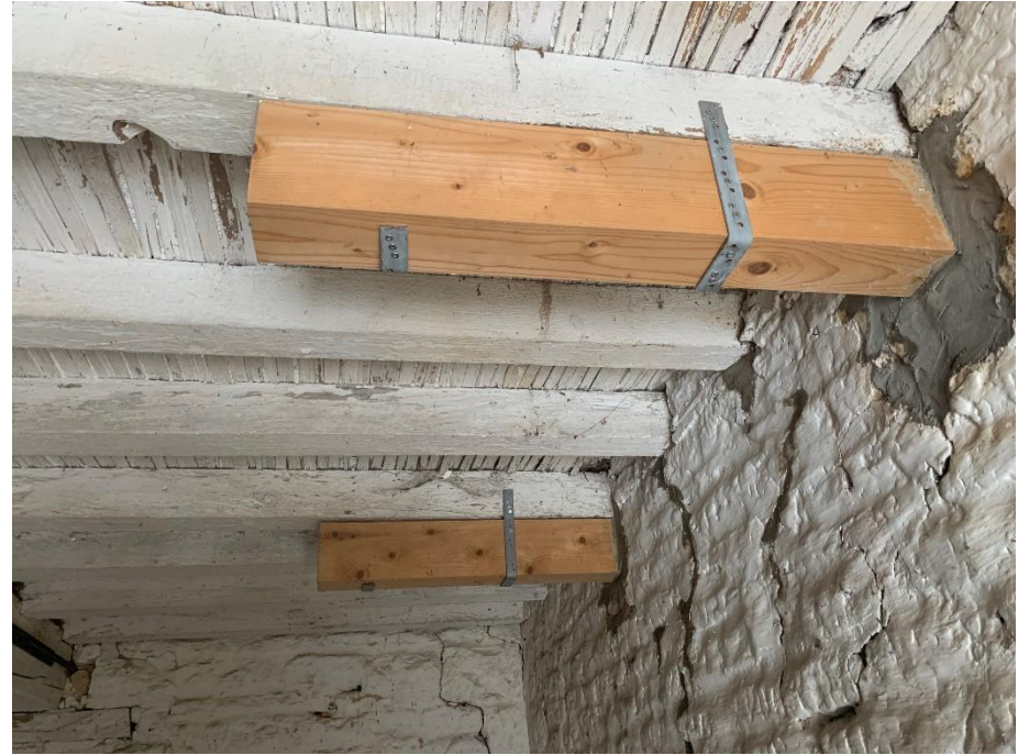
P20, left – Barn 3, detail of modern iron strap to beam. Laths laid over rafters are the base of the lime ash floor.
