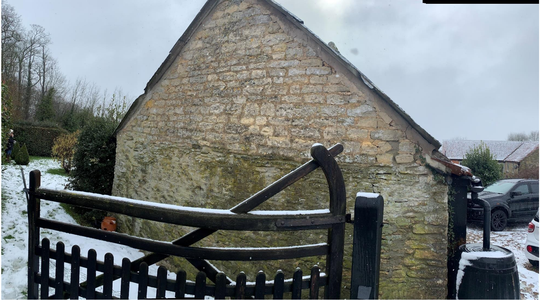
P10 – north elevation, shows the gable is a later overbuilding of an earlier structure. Note – to capture an image of the northerly gable, a panoramic photo was taken due to limited access - hence some distortion to the image.
