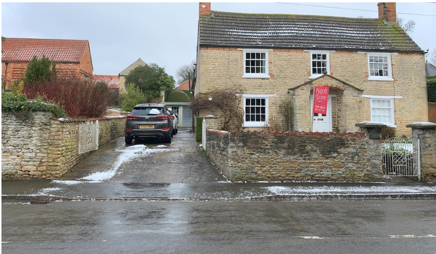
P1 – looking from Main Road towards Stone Barn, with Hill House on the right. Part of the south elevation of Stone Barn is seen with Hill House from the road.
