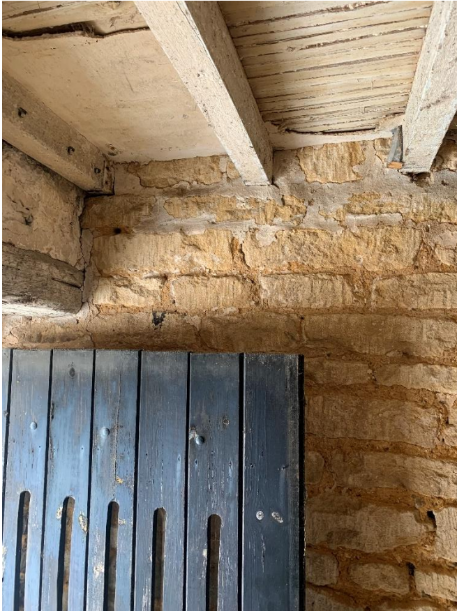
P17, left – lath and plaster between joists – lath above the joists form the base for a lime ash floor in Store 2 at first floor level.
