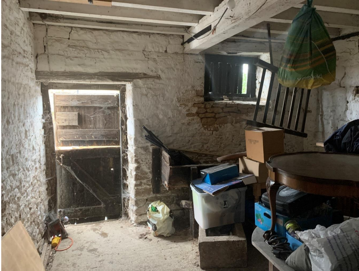
P22, left – stable door to Barn 3 with timber lintel above, feeding trough (below slatted breather vent).
