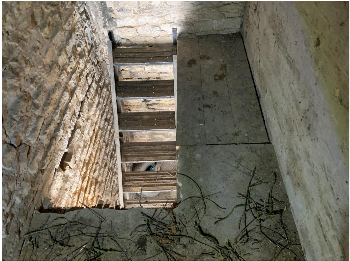
P17, left – lath and plaster between joists – lath above the joists form the base for a lime ash floor in Store 2 at first floor level.
