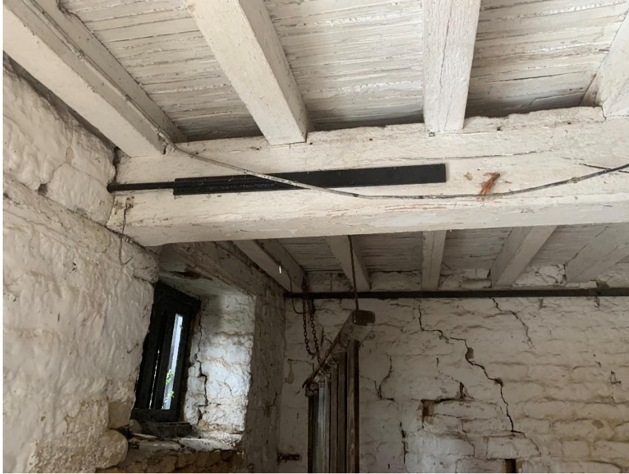
P20, left – Barn 3, detail of modern iron strap to beam. Laths laid over rafters are the base of the lime ash floor.
