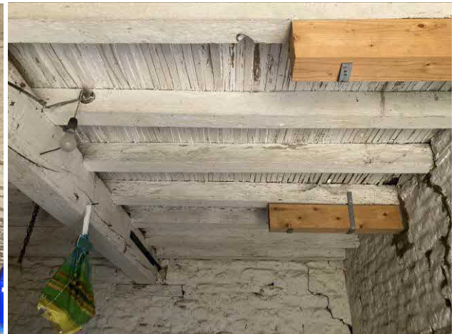
Exposed ceiling beams
