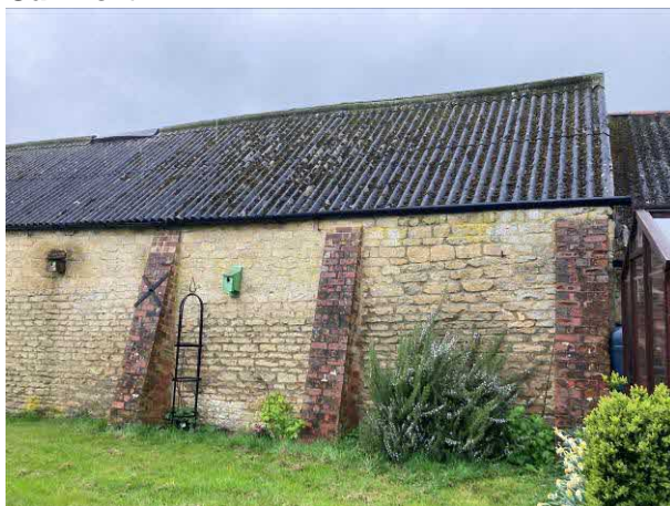
Rear face of car port
