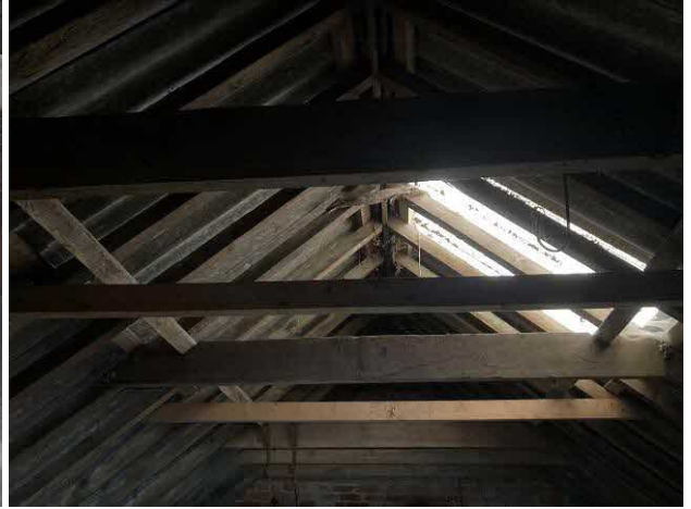
Underside of roof and light panels
