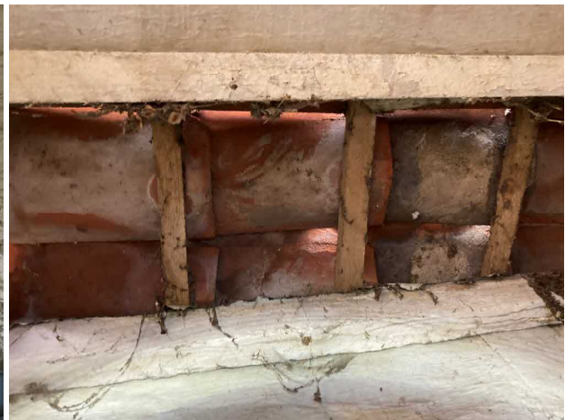
Underside of pantiles exposed
