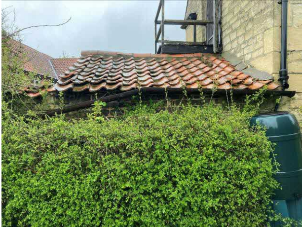
Rear roof of store
