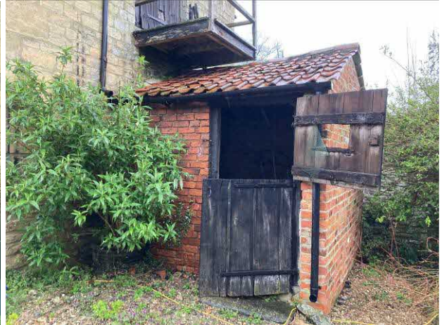
Front of store attached to south gable
