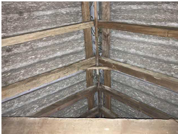
Underside of pitched roof
