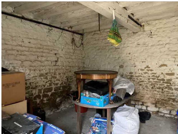
Interior ground floor of barn
