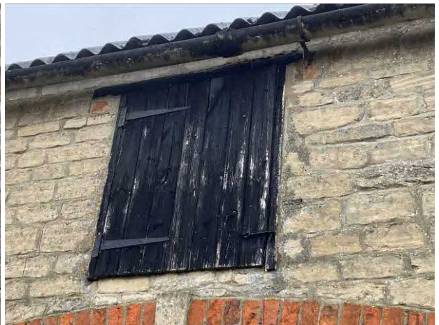
Boarded windows to the granary room
