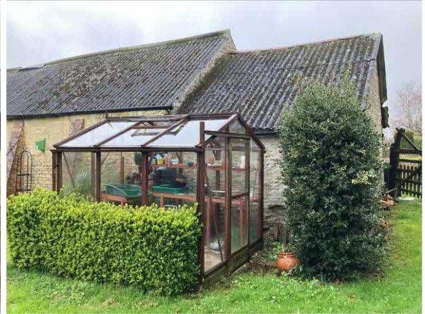
Rear of garage
