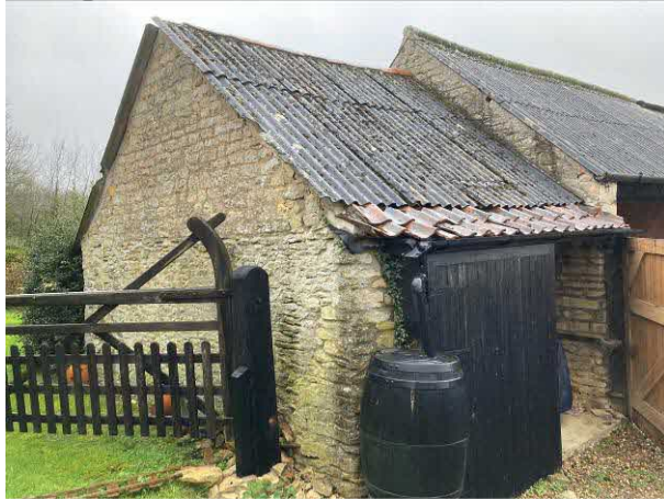
Front and north gable end
