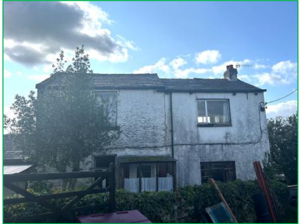
The east elevation of the cottage
