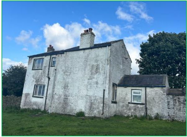
The west elevation of the cottage
