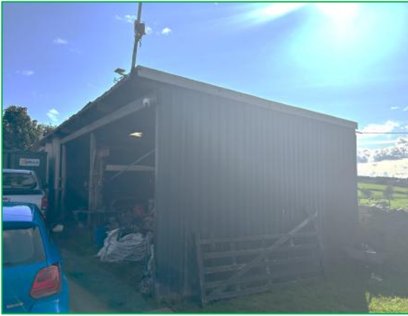
The northeast elevation of Outbuilding 1
