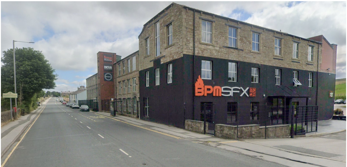
Oak Mill, Manchester Road, Dunnockshaw, Burnley
