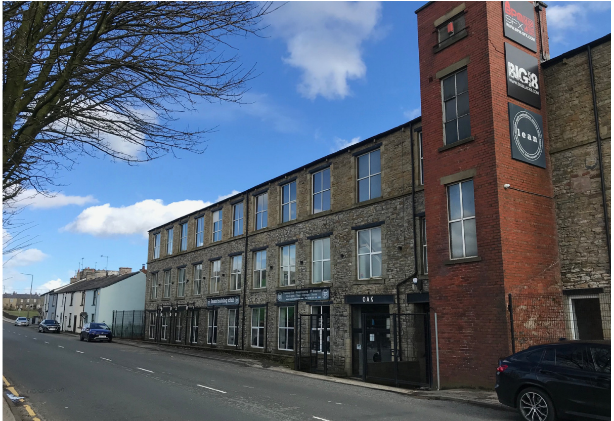
Ground floor indicated to become part of existing commercial business. Any LEAN signage to be removed
