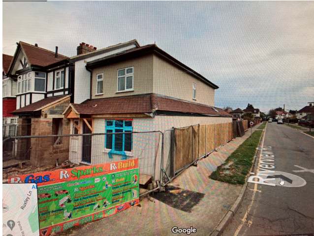
View from side showing front of 135 and 135a
