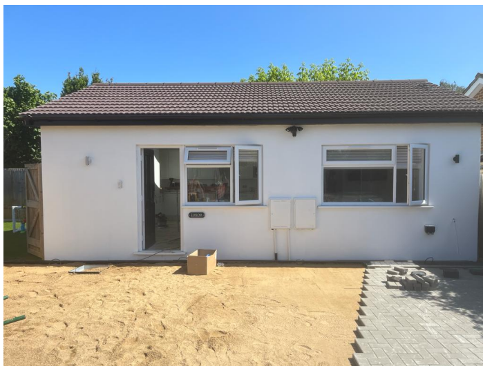
Front of garage, amended for use in association with 135 Riverview road, showing security lights, meter and car power charger.
