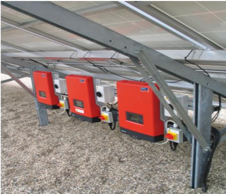
Below is an image of the inverter mounting and location behind the panel array
