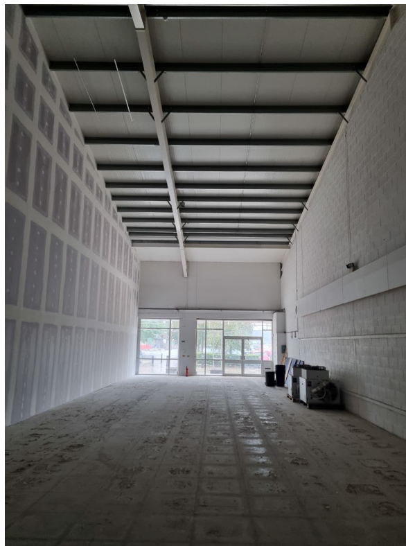
VIEW FROM INSIDE THE EXISTING UNIT OF THE SHOPFLOOR
