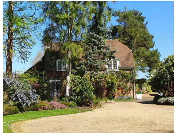
Plate 16. Converted coach house to the north
