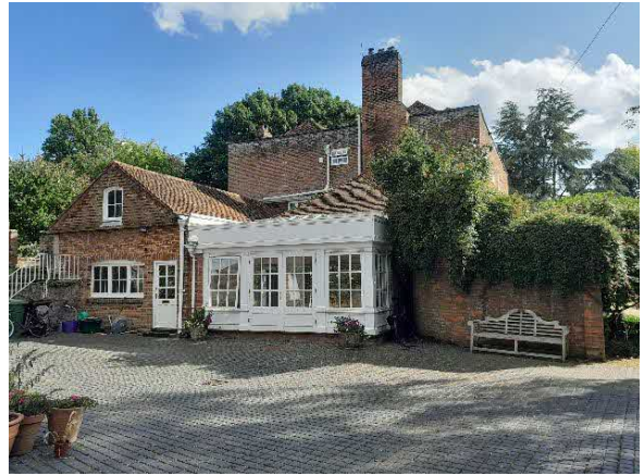
Plate 14. The Postern (north facing elevation)
