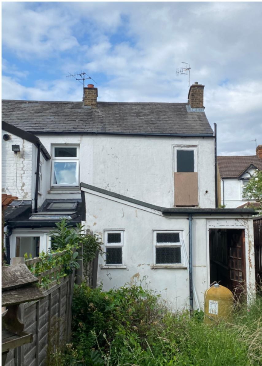
Figure 2: Site Photograph (prior to changes)
