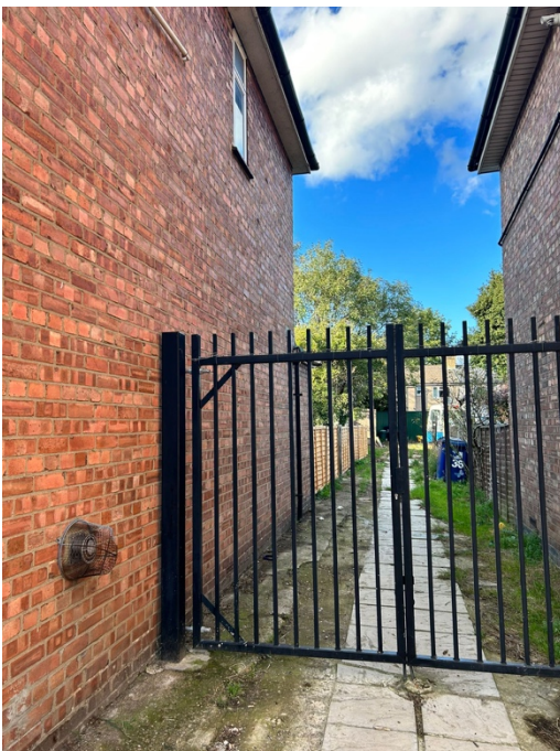
36 Sunningdale Avenue - DRIVEWAY
