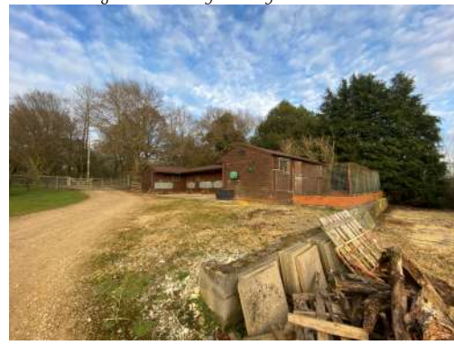
Figure 4 - View of stables from the south.
