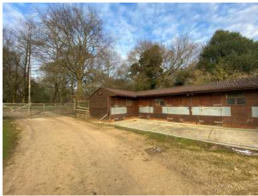
Figure 3 - View of stables from the south.
