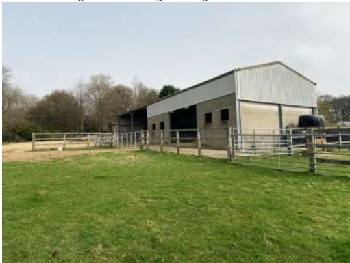
Figure 5 - View of existing barn beside stables.
