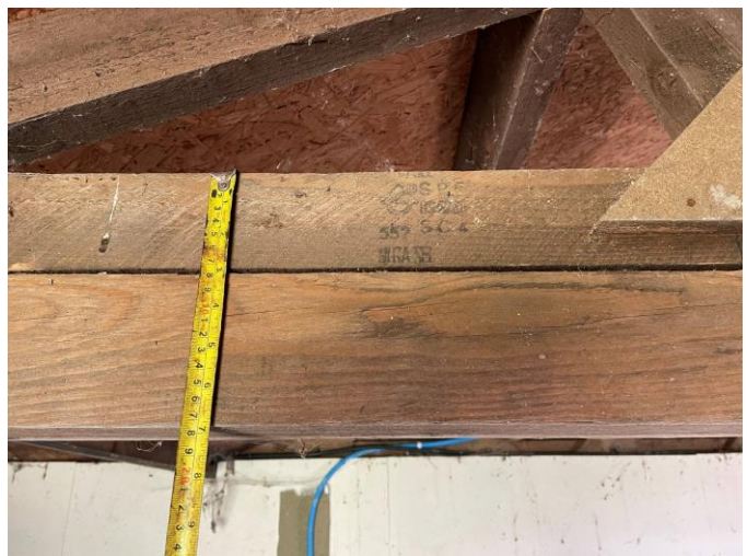
16. Small section roof trusses (75mm) and supporting joist
