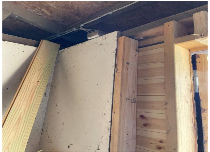
18. Replacement timber wall studding
