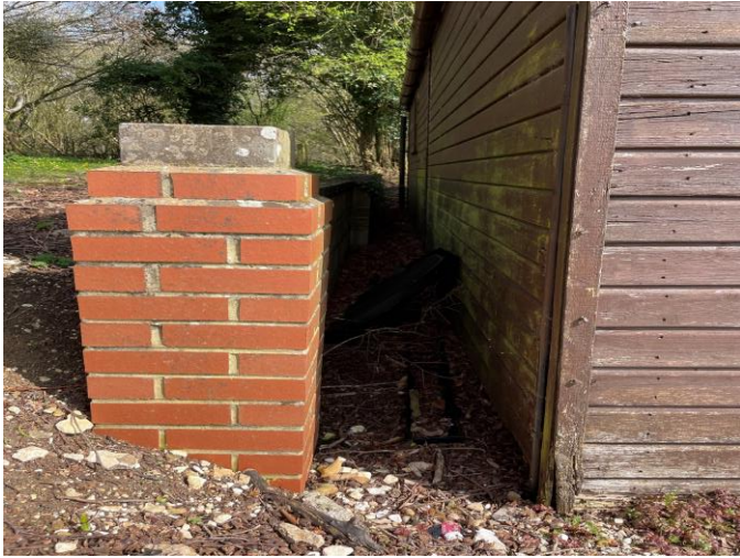
9. Retaining wall to north elevation
