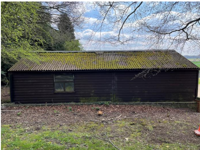
3. North Elevation. Note the profiled roof sheets and block plinth
