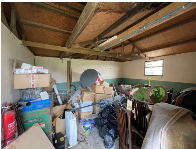
15. Lightweight timber roof structure and wall boarding
