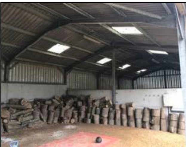
Image 19: An internal view of the north portion of B2, facing south.
