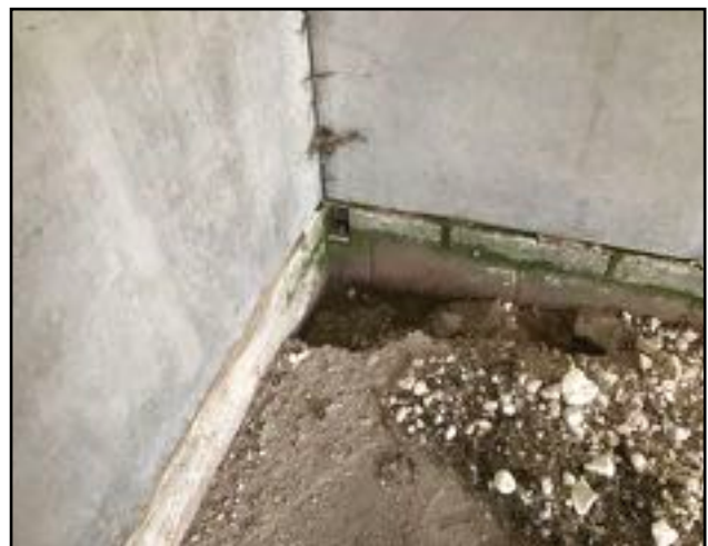
Image 20: Digging was found in the south portion of B2, and various animal droppings were found nearby.
