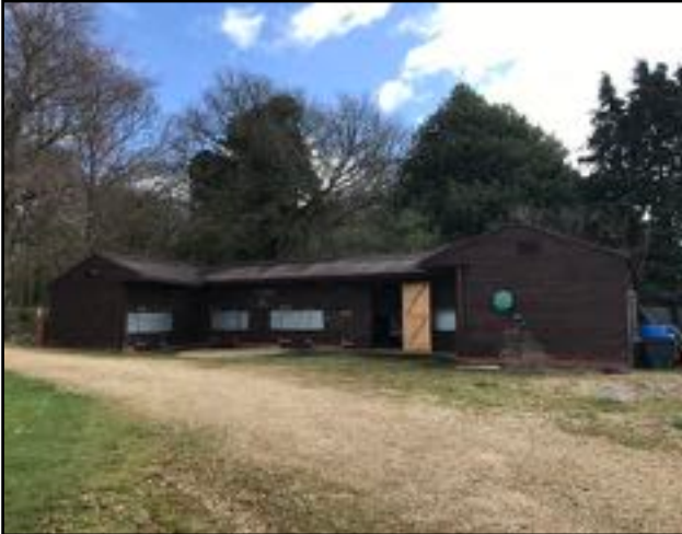
Image 1: The front (west) elevation of B1.
