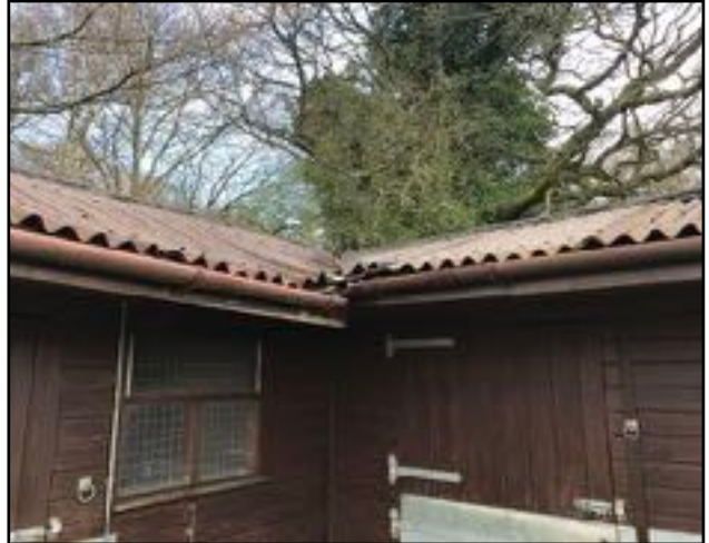
Image 2: A view of the roof structure on B1.
