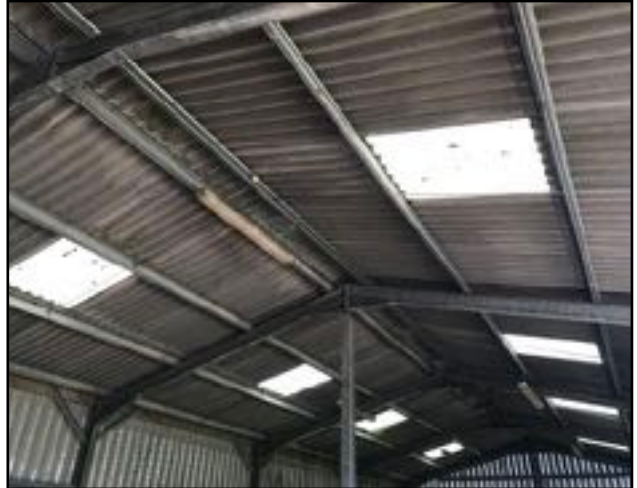
Image 16: A view of the underside of the roof of B2.
