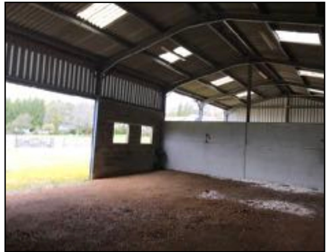
Image 18: An internal view of B2, facing northwest.
