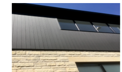
Composite Cladding by Hyperion Fire Rating - Class D Carbon Footprint - 69% lower than timber Recycled Materials - 90% recycled
