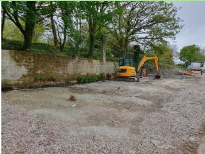
T3, T2 and T1 behind retaining wall
