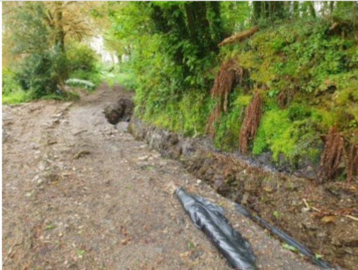
Trench on western edge of driveway
