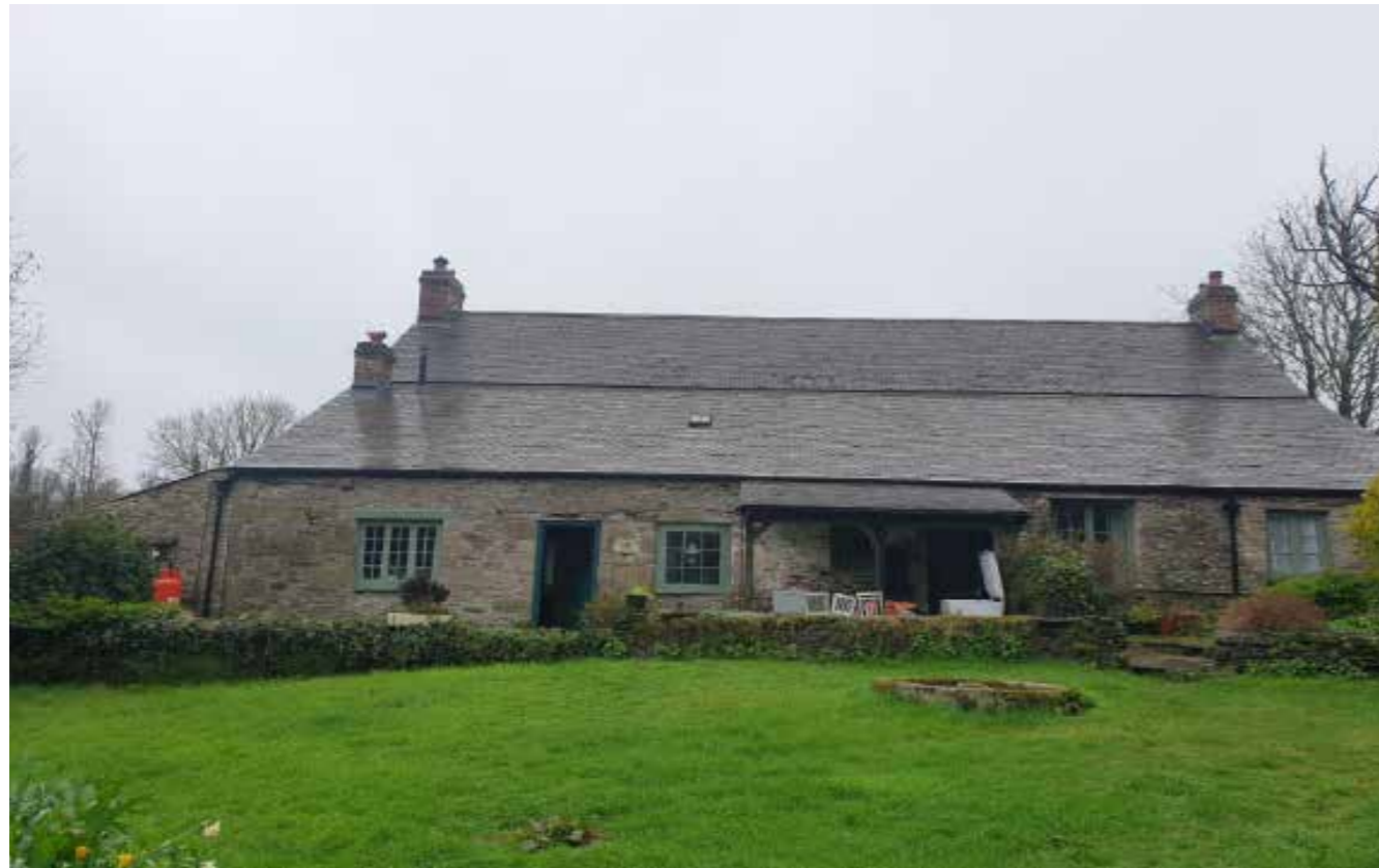
Image 4. Rear Elevation North
