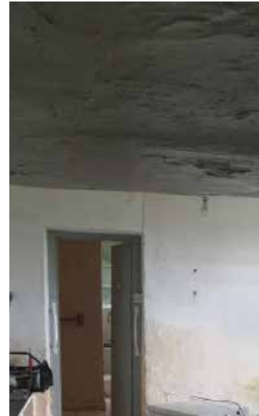
Image 22. Internal ground ceilings
