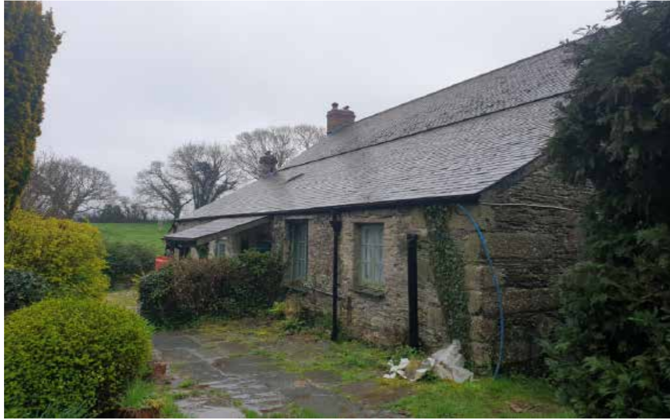
Image 2. Existing Catslide Roof North
