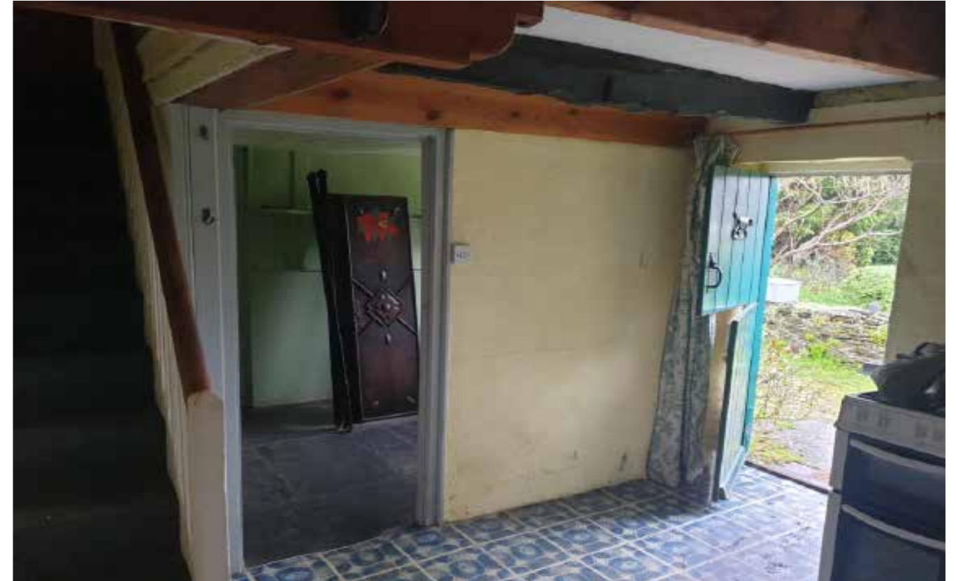
Image 11. Internal ground ceilings
