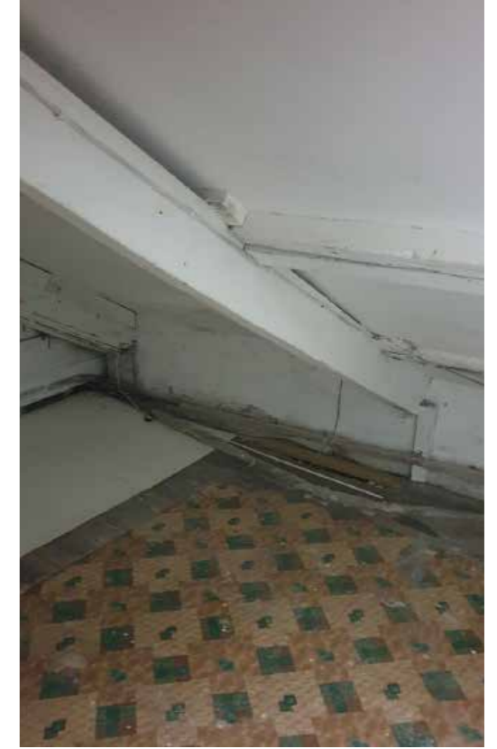
Image 18. Internal catslide roof
