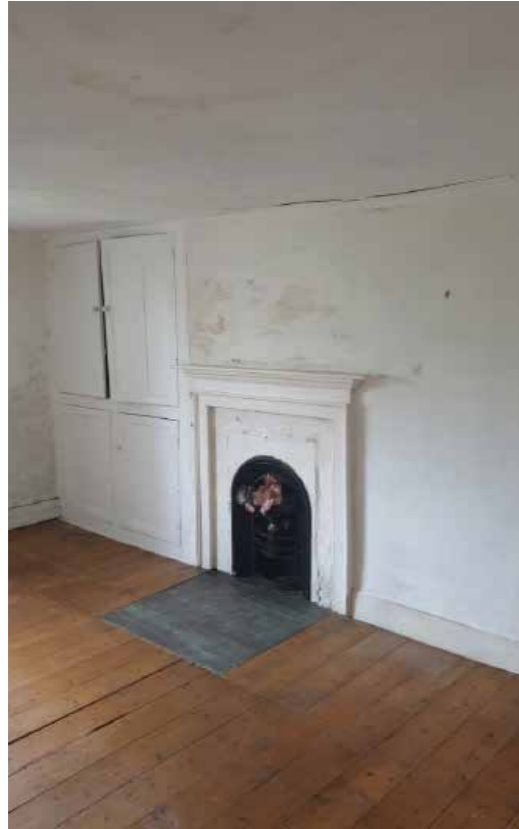
Image 14. Southern slate floors. Fireplace SW Bedroom
