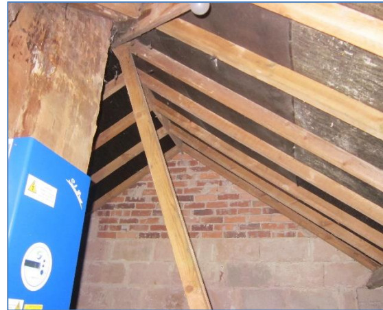
Example void interior, dividing wall between semi-detached houses.
