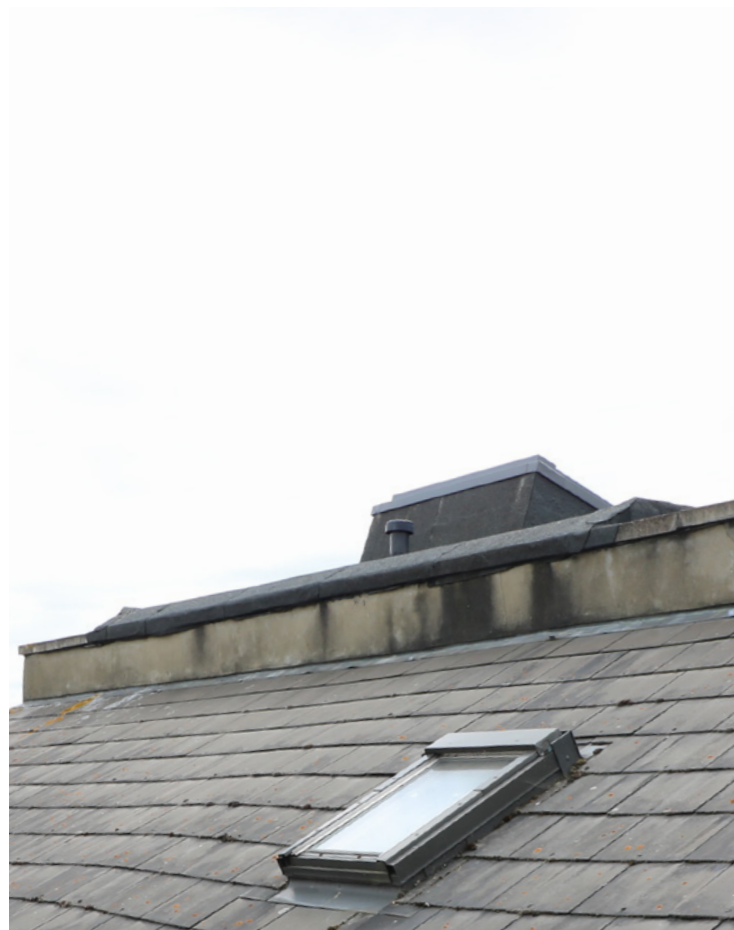
Extent of No. 38 Beckwith Road's roof extension
