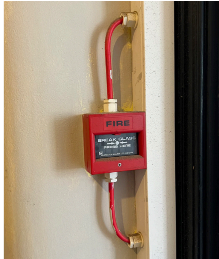
Multi-zone fire alarm system and 'break glass' fire alarms points
