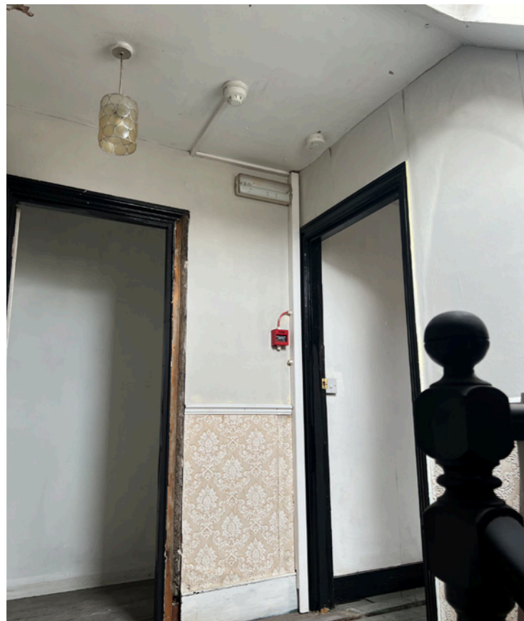
Emergency lighting and fire alarms in the 1st floor and 2nd floor hallways and landings
