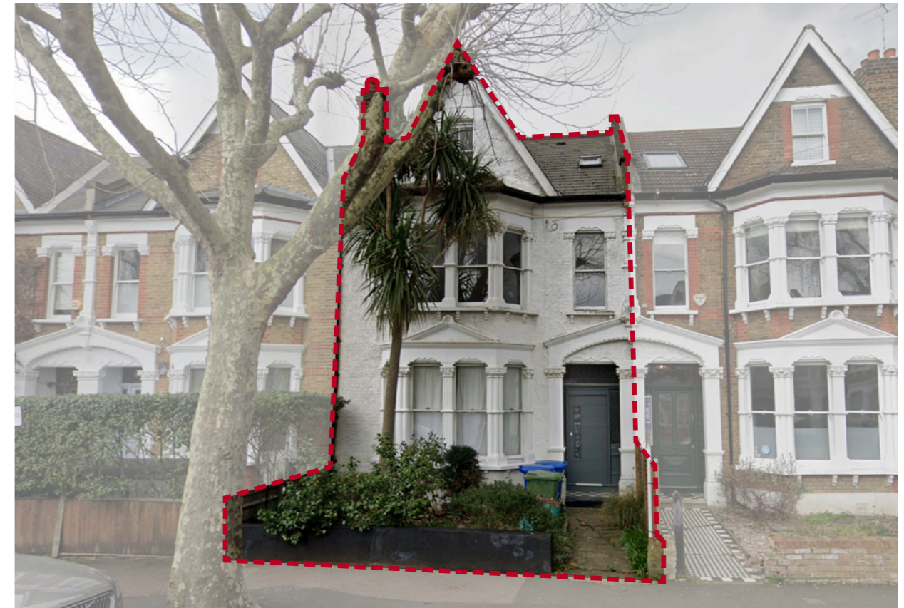
View of Beckwith Road street elevation
