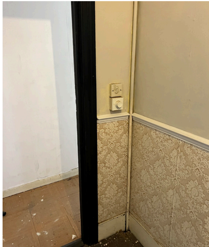
Push button light switches in the 1st floor and 2nd floor hallways and landings
