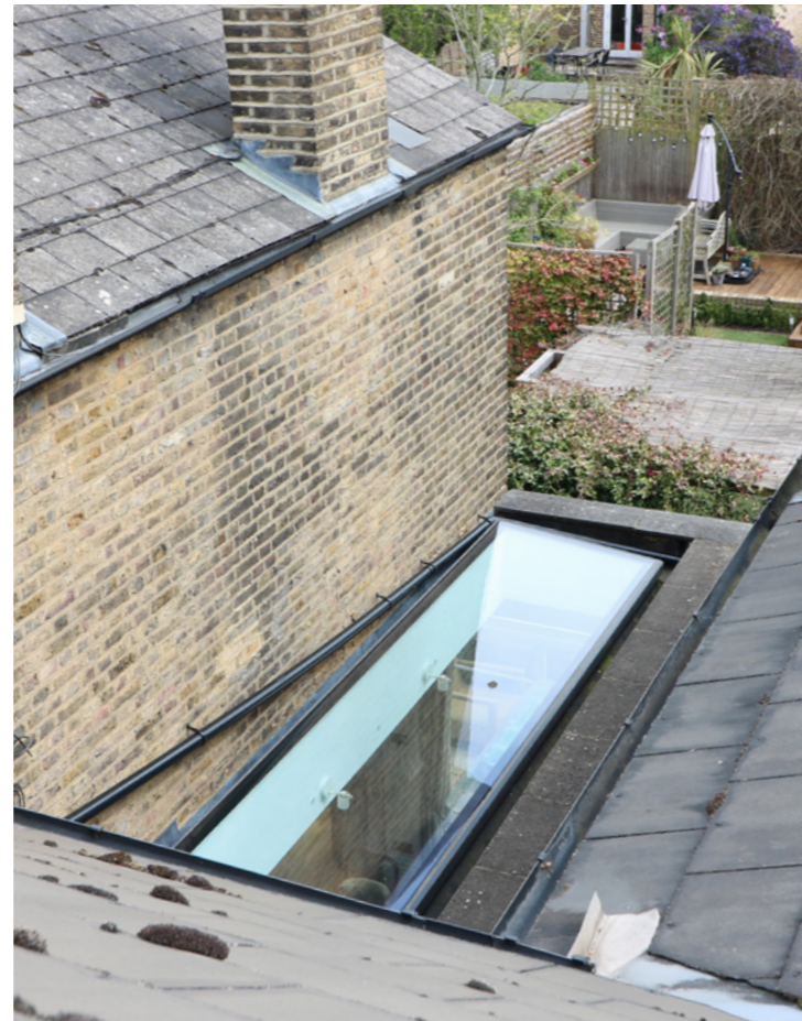
Roof of No. 42 Beckwith Road's side extension
