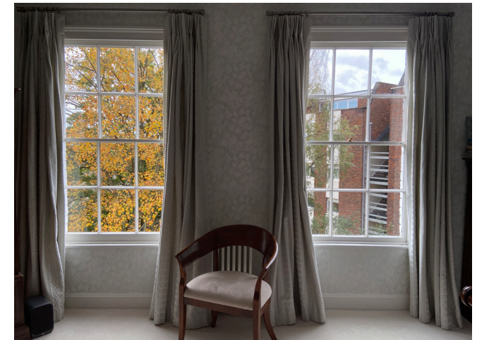
Existing sash windows at Second floor - to be replaced
