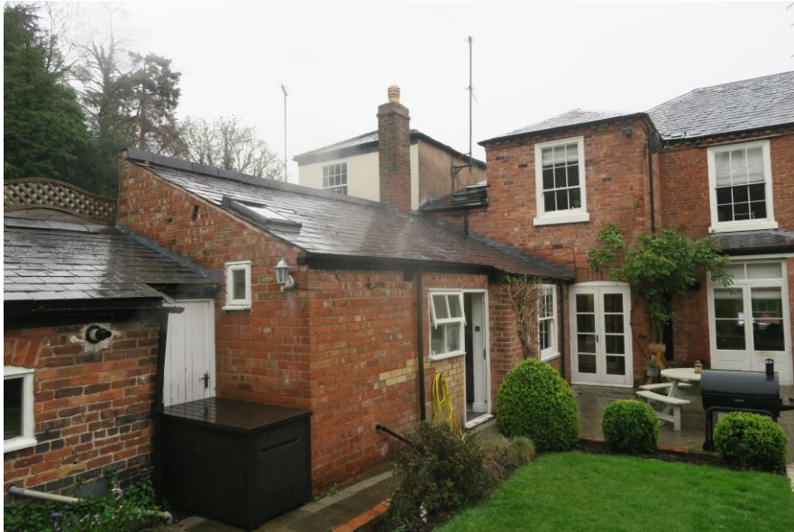
Rear Elevation of the existing dwelling
