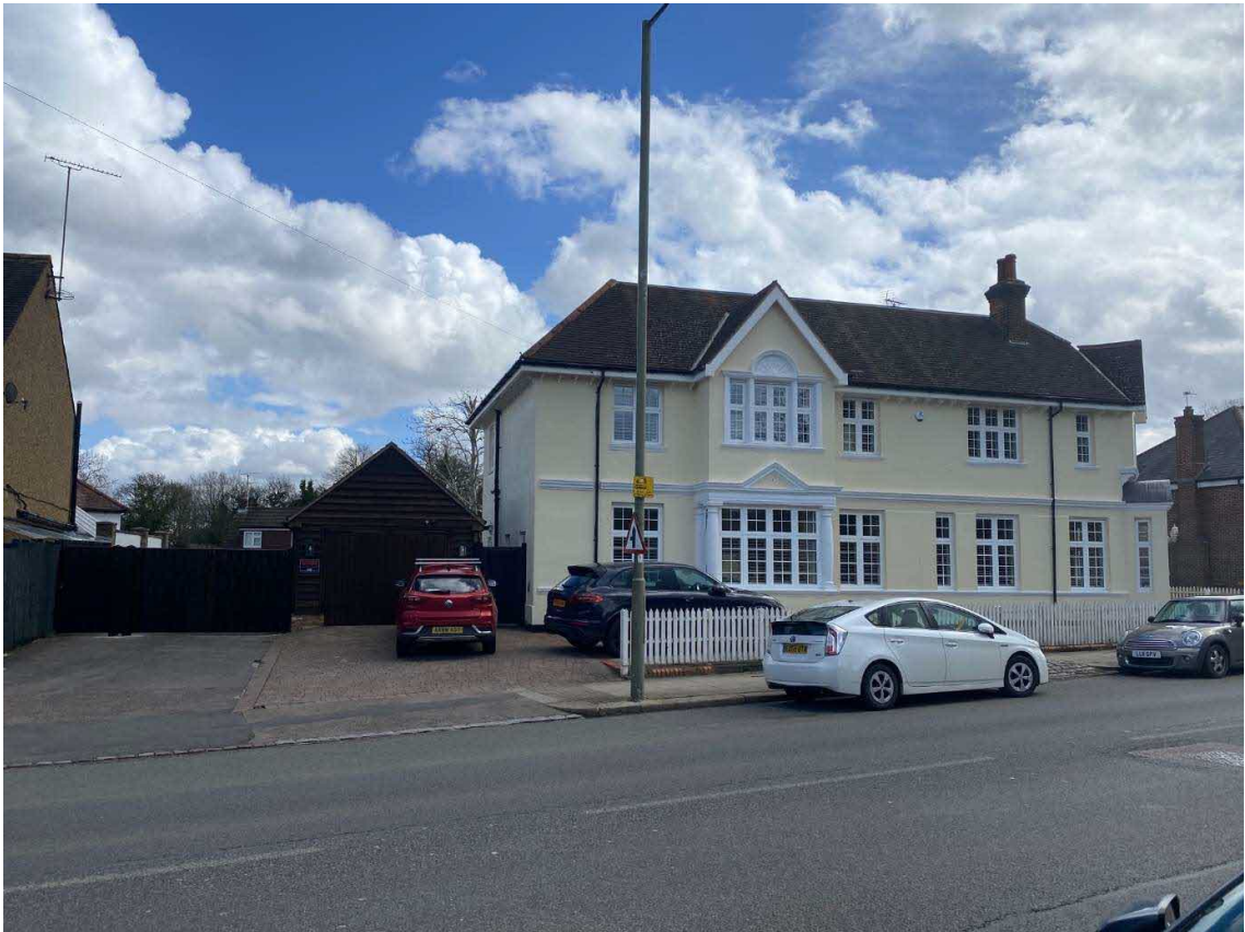
Current view showing 12 and 14 together with existing crossover and store to be demolished
