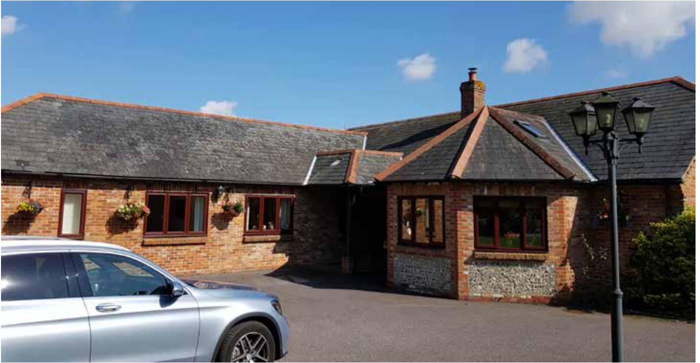
Photograph No. 1 - Northern aspect of building B1.
