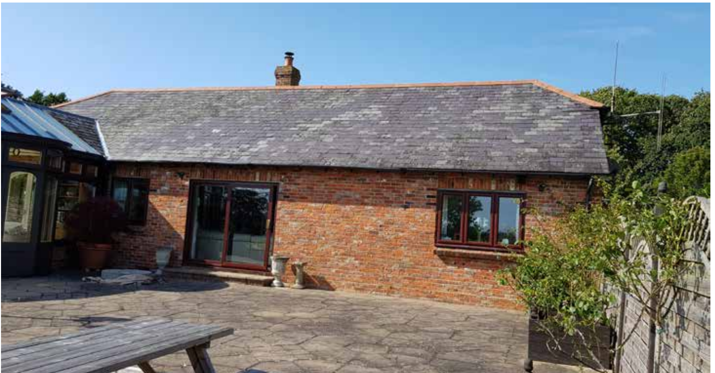
Photograph No. 2 - Southern aspect of building B1. The proposed extension footprint will lie solely within the existing hard ground.
