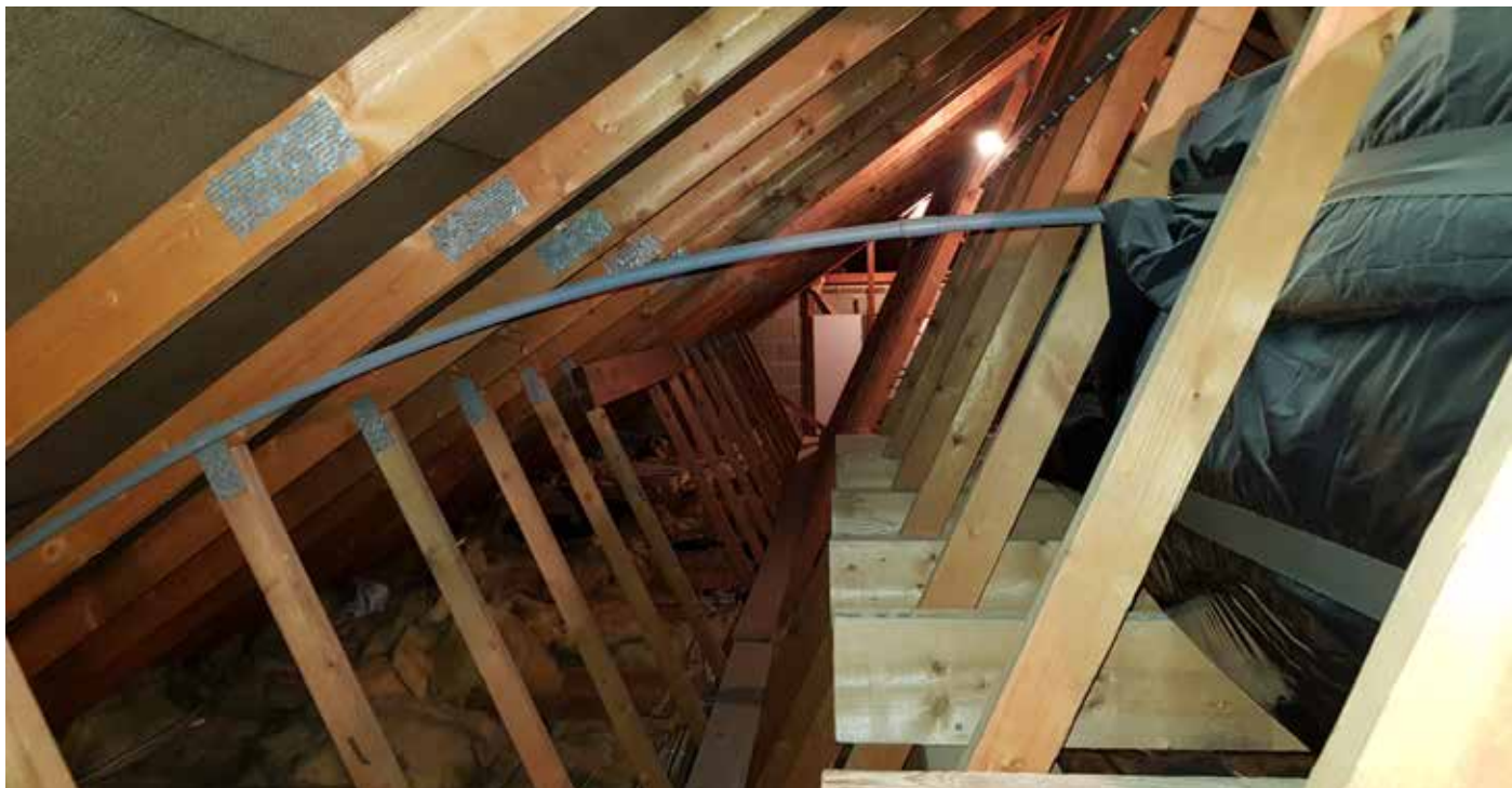
Photograph No. 3 - Internal view of the loft space.
