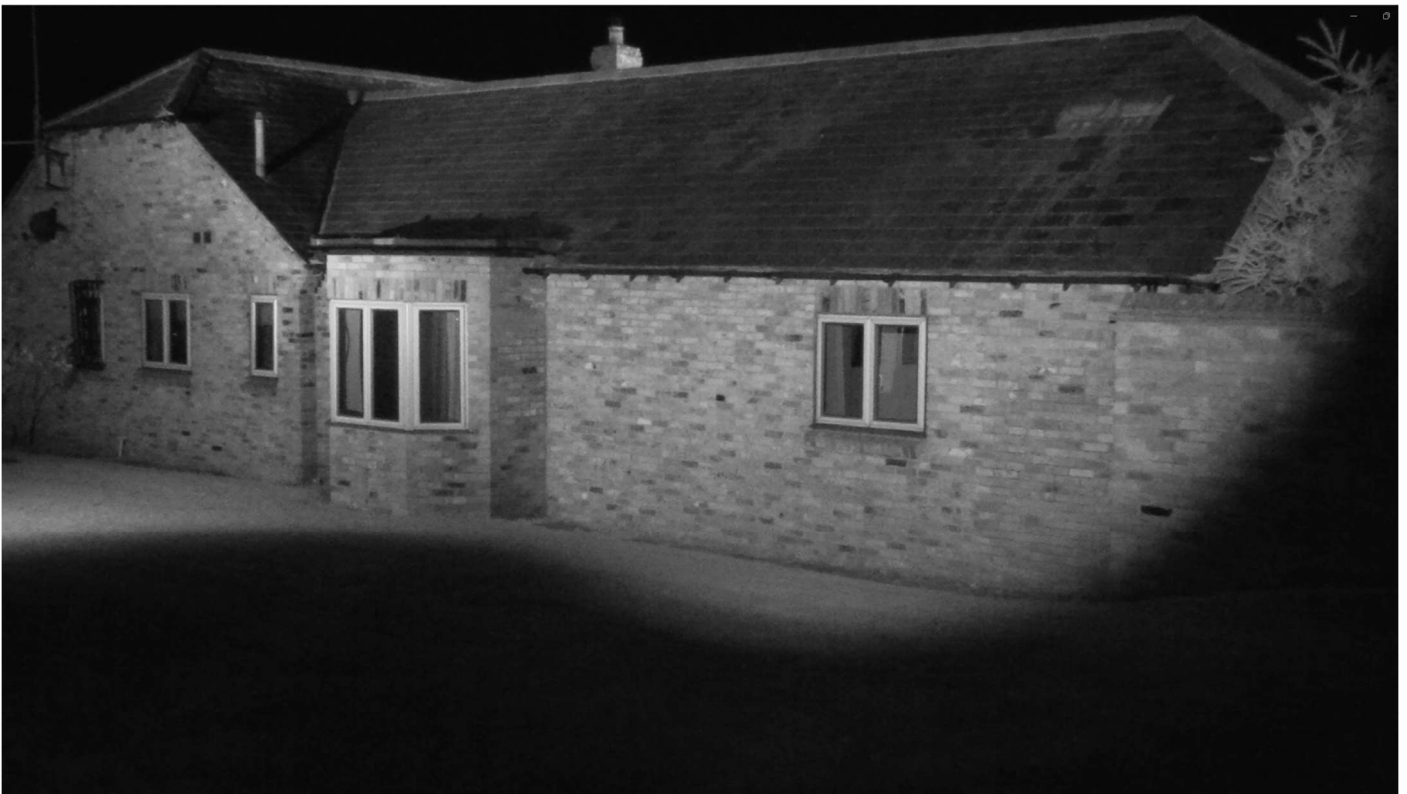
Photo 6 – Example of NVA Footage from the east, end of survey.
