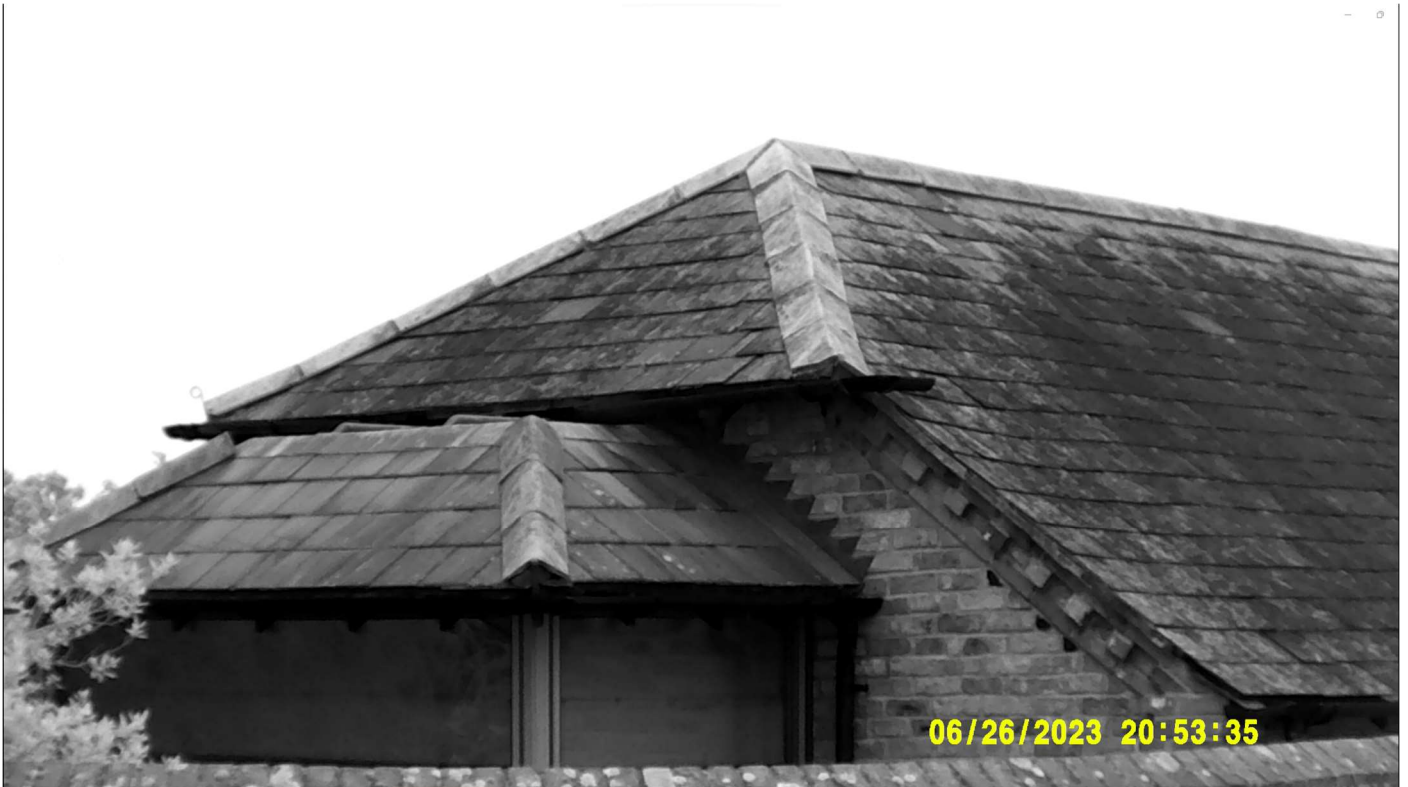
Photo 3 – Example of NVA Footage from the north (Whisker), start of survey.
