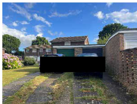
Fig.5 – Neighbouring garages east of the host garage
