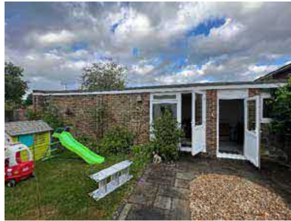
Fig.8 – View looking E to the existing outbuilding from the conservatory
