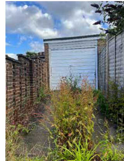
Fig.6 – Site garage and parking space in front
