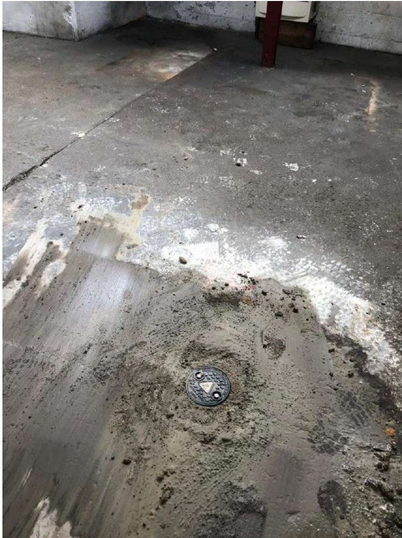
Photo 11 – Showing the borehole installed with monitoring wells and borehole cover
