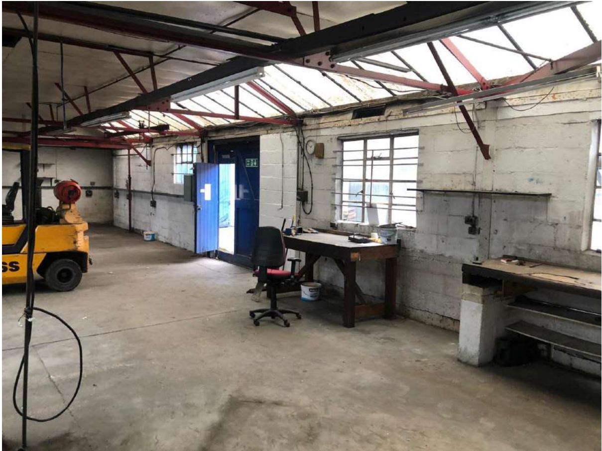
Photo 5 – Showing inside the building (114-116 Hythe Street)
