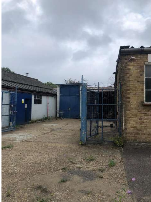
Photo 3 – Showing the concrete track between the 2 buildings
