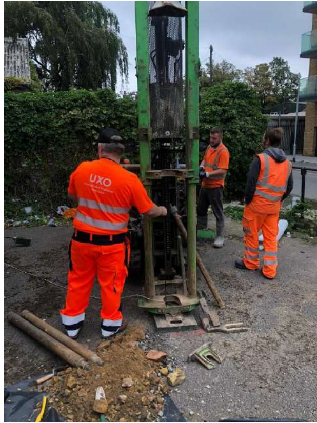
Photo 7 – Showing the UXO Detection Engineer clearing the borehole
