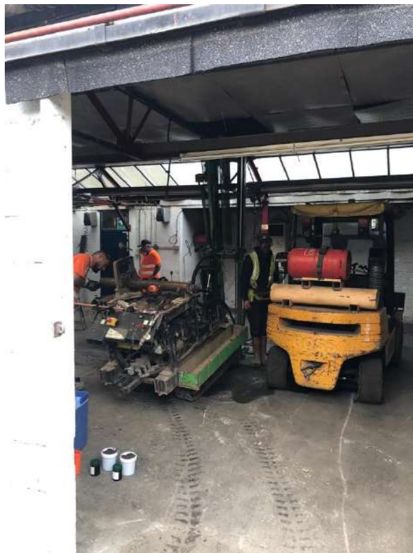
Photo 6 – Showing the rig set up at WS01
