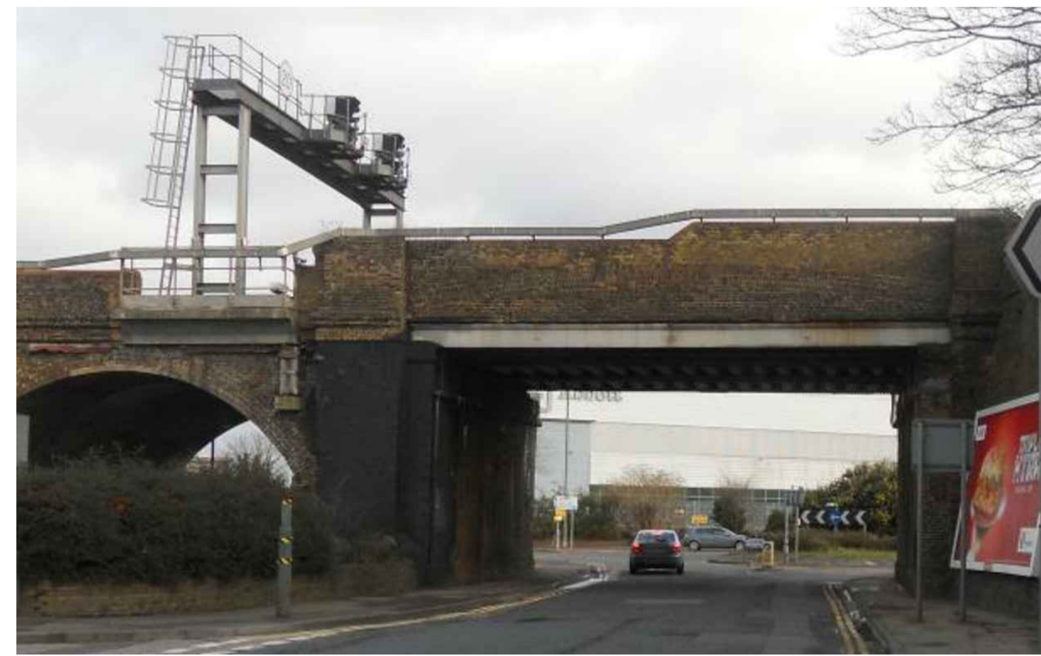
View Looking North
