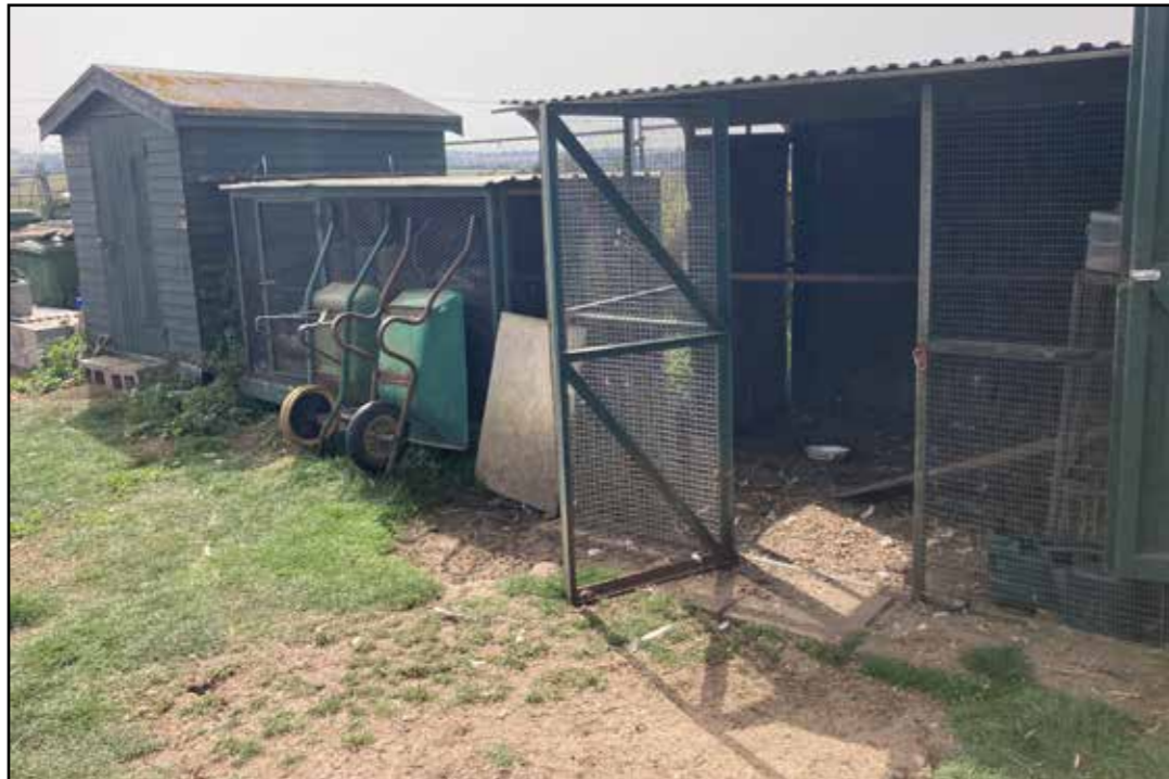
Structures that will be demolished include sheds and chicken coops. There are no features suitable for roosting bats.
