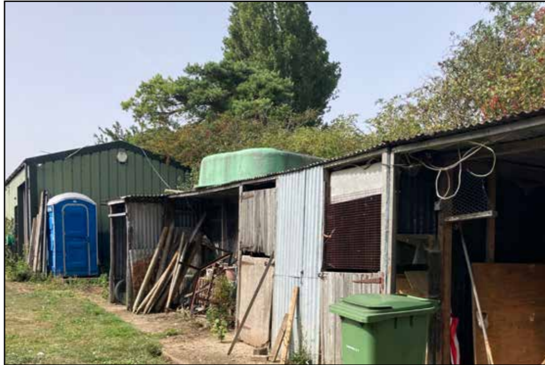
Structures that will be demolished include various outbuildings. There are no features suitable for roosting bats. Some outbuildings could support nesting birds. A mature hedge that is dominated by hawthorn with some ash, elder and fruit trees is present along the northern boundary.
