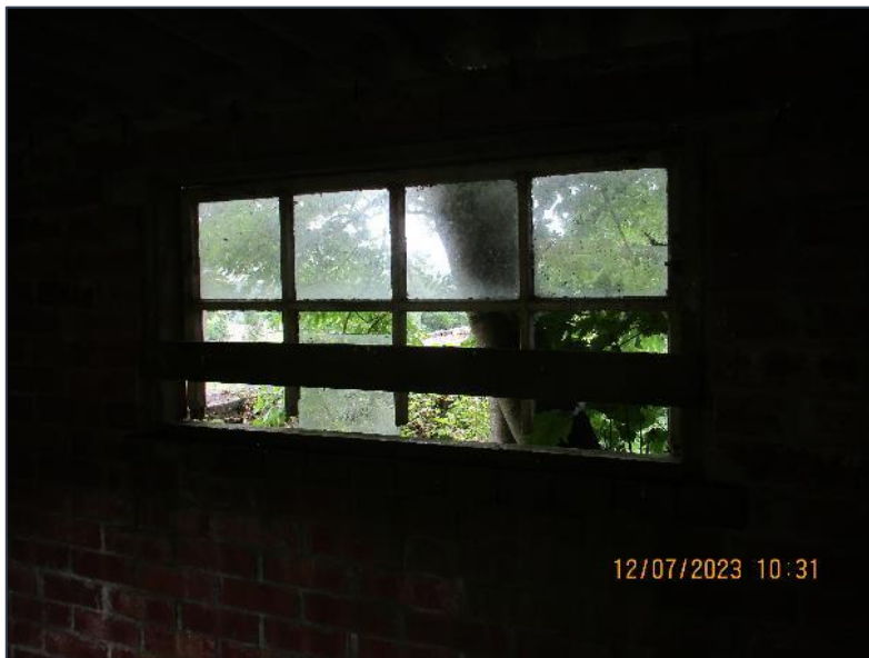
Photograph E Window to south elevation.
