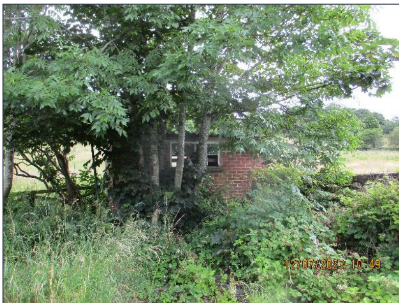
Photograph C South elevation of building.
