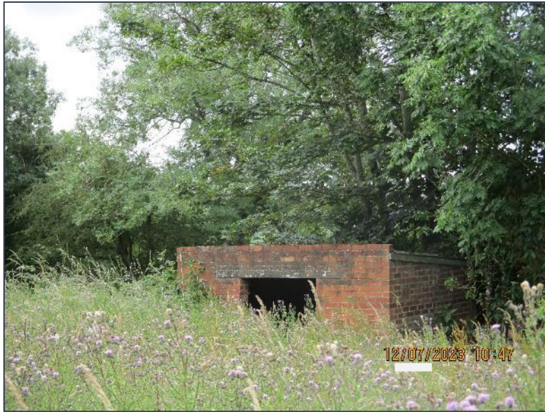
Photograph A Northern elevation of building.
