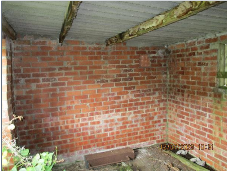
Photograph D Interior of building.
