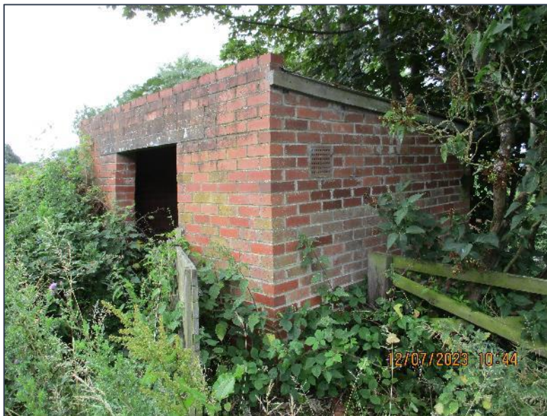
Photograph B North and west elevations of building.
