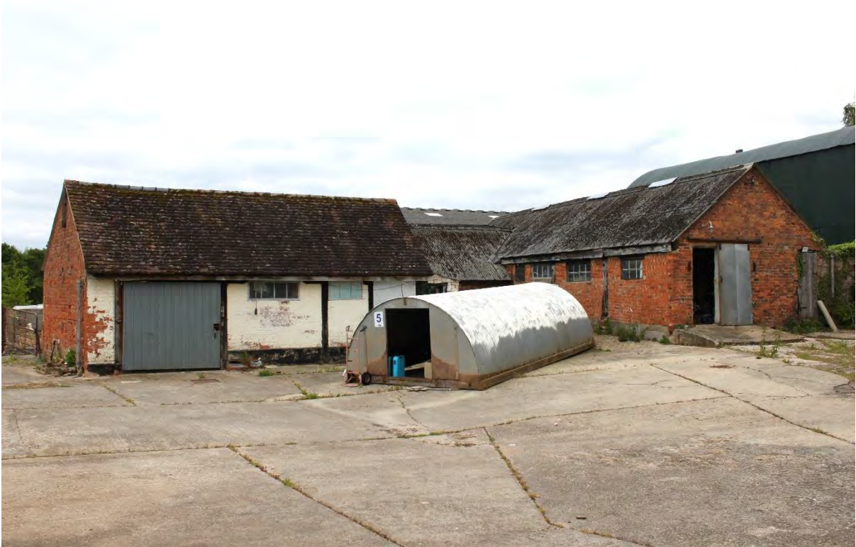
Figure 34: Plate 21 Former farmyard, looking northwest
