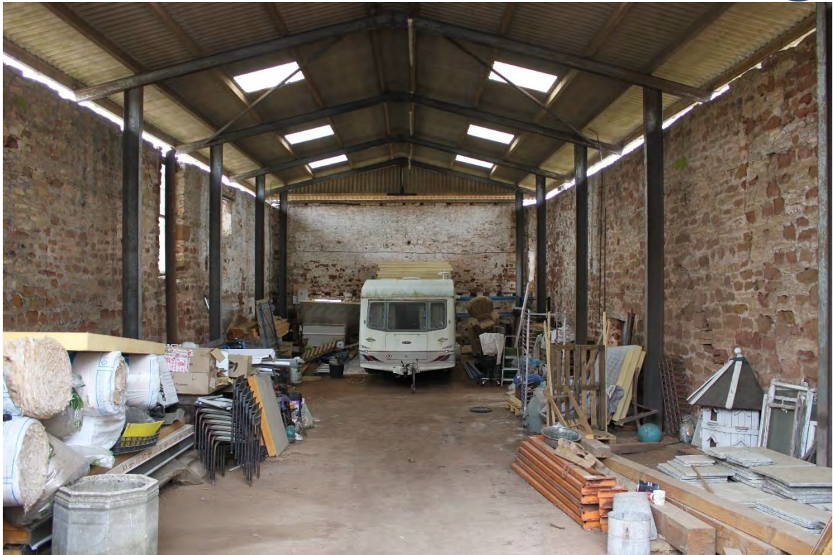
Figure 47: Plate 34 The building, interior, looking south
