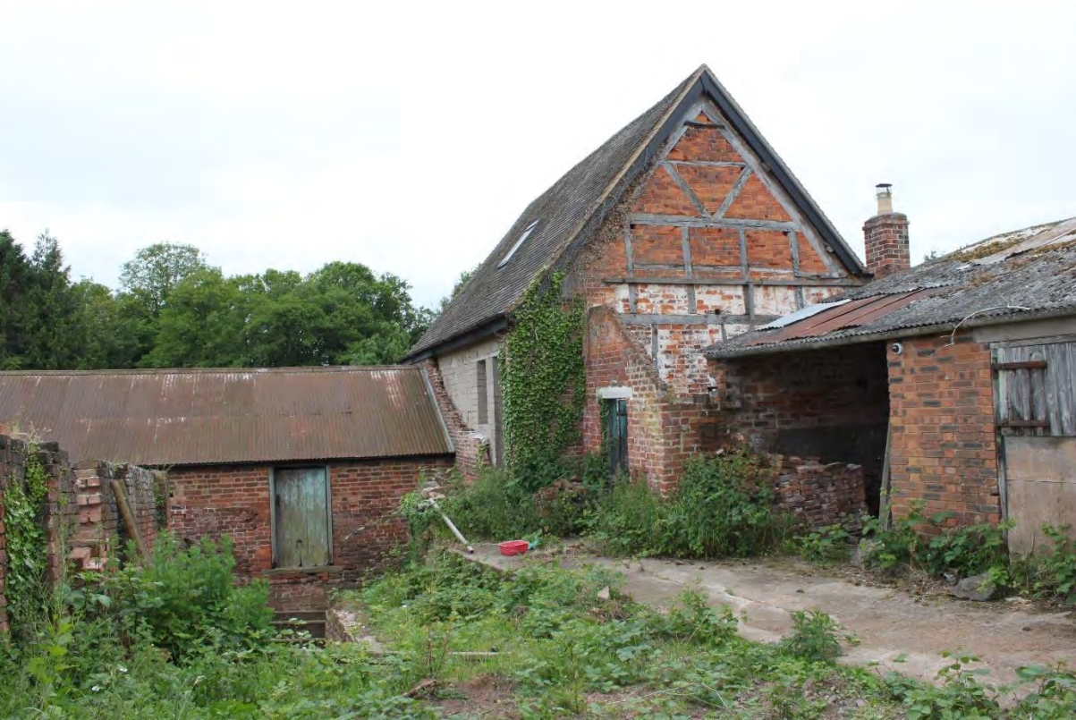
Figure 28: Plate 15 View to the structure understood to include the former Blowing House, looking southwest
