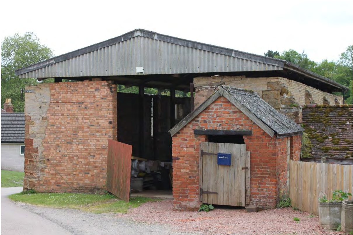
Figure 44: Plate 31 The building, view to the north elevation, looking southeast
