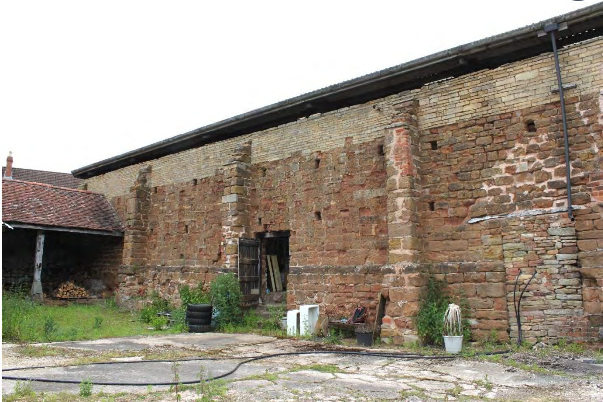
Figure 18: Plate 5 The building, view to the west elevation, looking northeast
