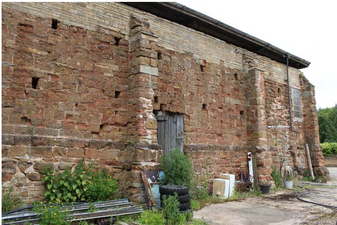
Figure 21: Plate 8 The building, view to the west elevation, looking southeast
