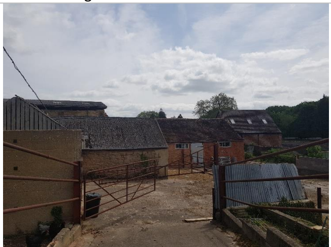
Other buildings adjacent to the site.
