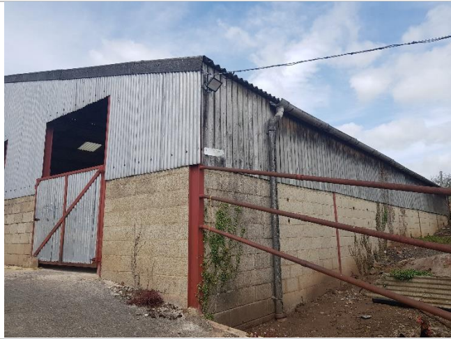
Exterior of the barn. South facing gable pictured.
