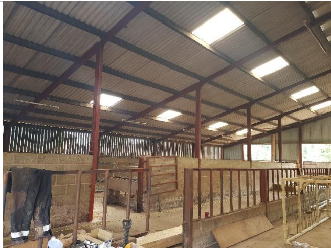
Interior of barn.
