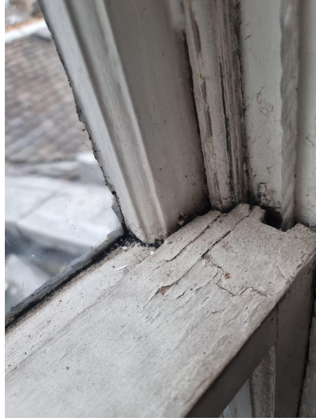
Failing seals around the glass and woodwork at the joints appears to be splitting and rotting under the paintwork.
