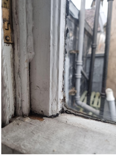
Failing seals around the glass and woodwork at the joints appears to be splitting and rotting under the paintwork.
