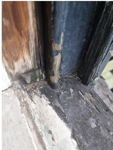
Rotting parting beads, sills and casement woodwork.
