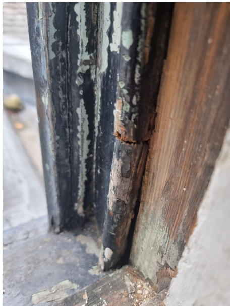
Rotting parting beads, sills and casement woodwork.
