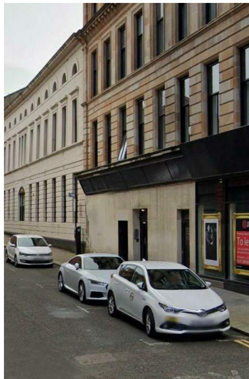
3. Walls Street frontage
