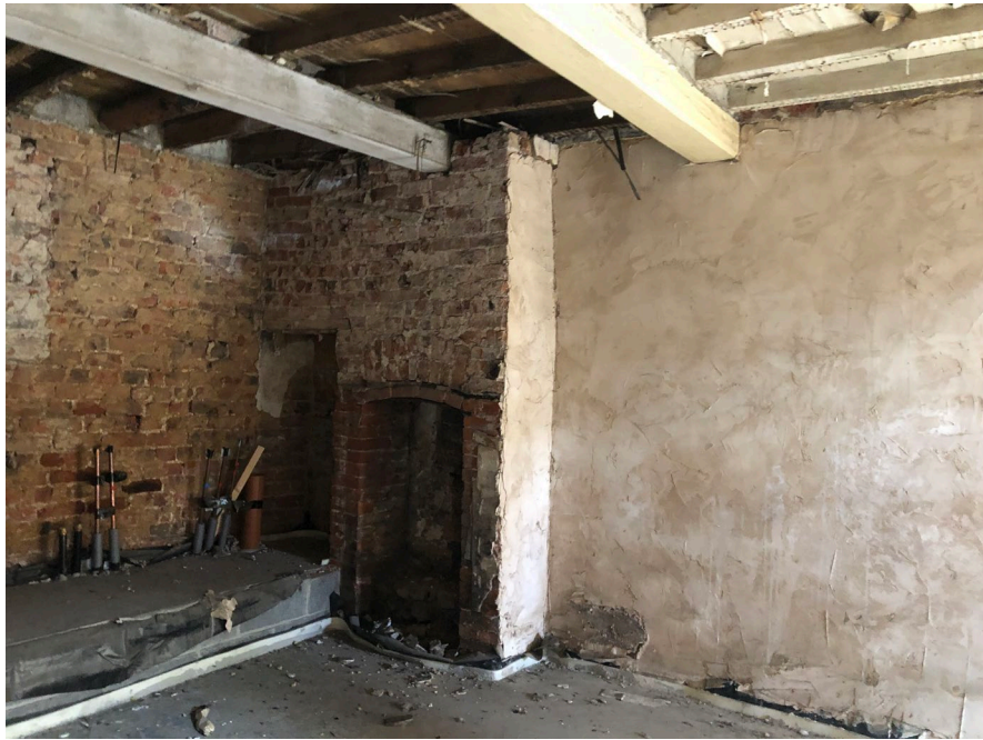
Photo 9: Chimney breast to be retained
