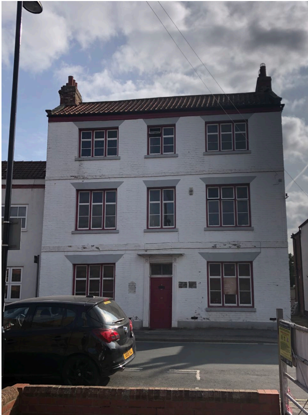
Photo 1: The front (west) elevation
