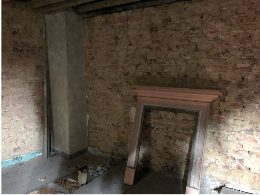
Photo 8: Fire surround in storage
