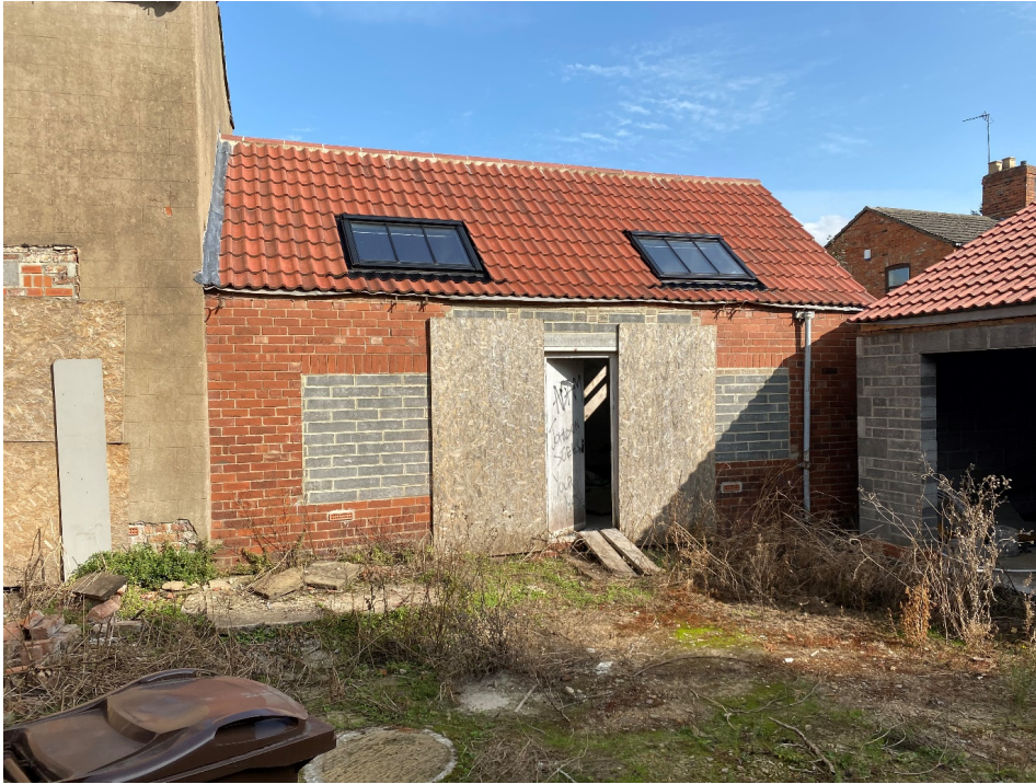
Photo 4: Modern, rear extension
