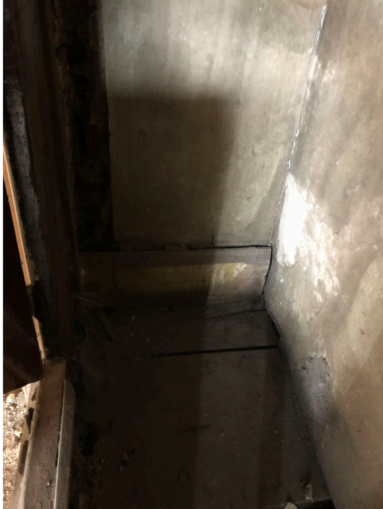
Photo 11: Surviving skirting on first floor
