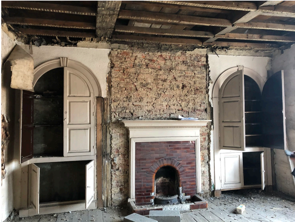
Photo 12: Surviving cupboards on first floor
