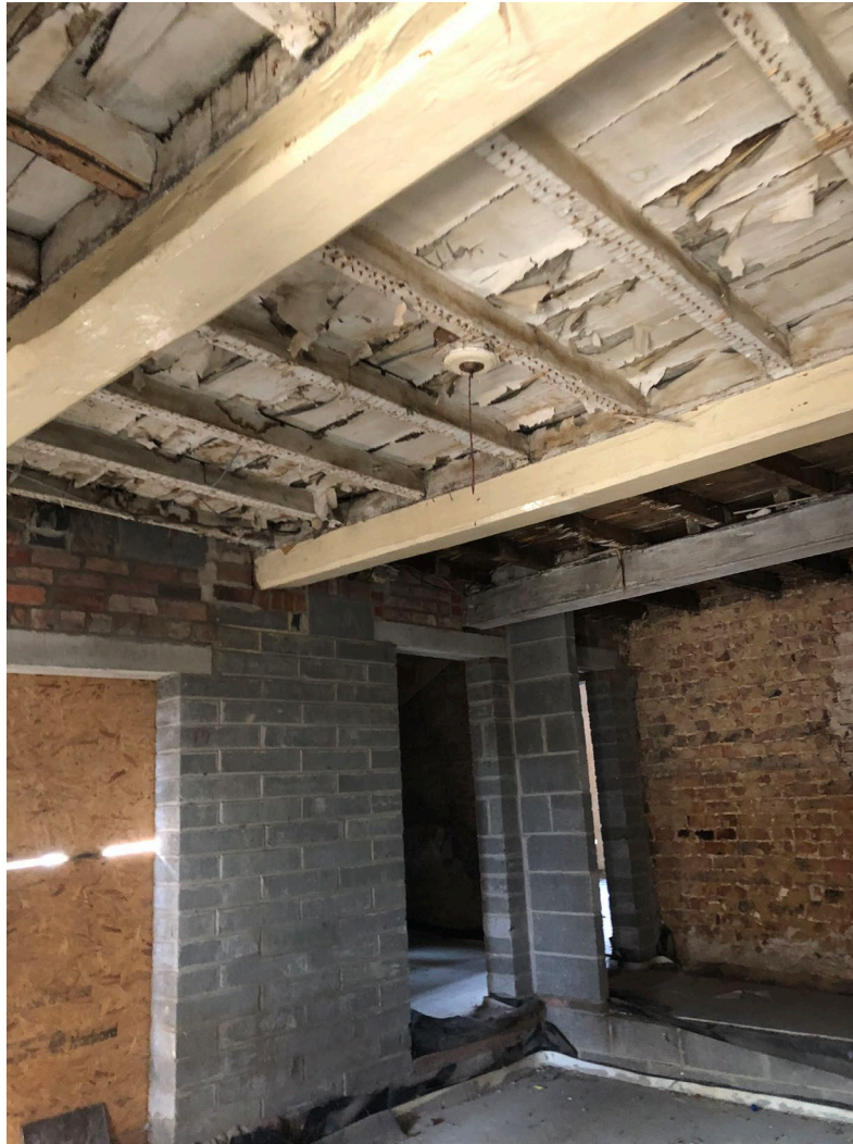
Photo 10: Painted underside of first floor
