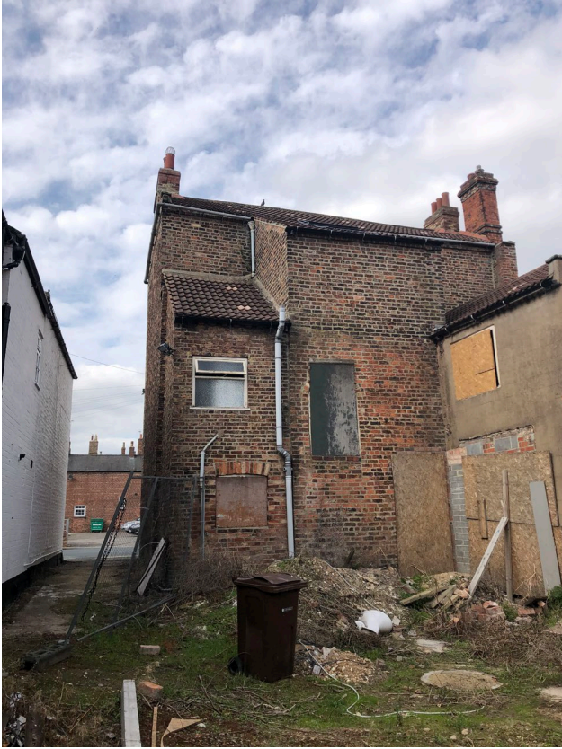
Photo 2: Rear (east) elevation of the frontage building
