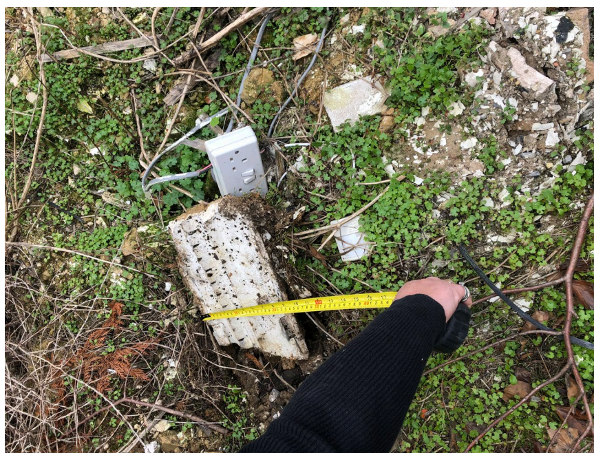
Photo 5: Cornice fragment retrieved from spoil heap
