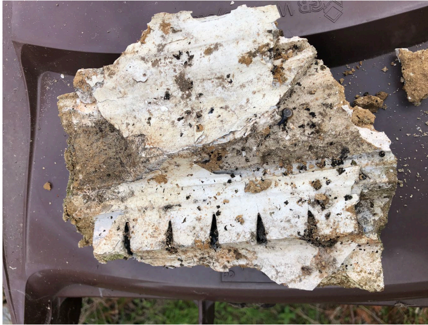
Photo 6: Fragment of cornice found in spoilheap
