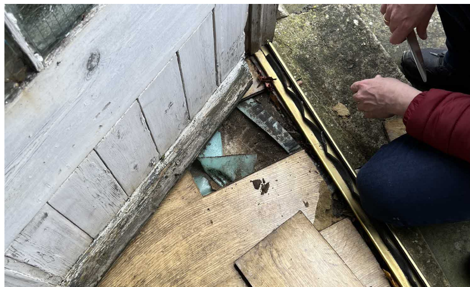
Fig 20. Concrete screed and laminate floor covering
