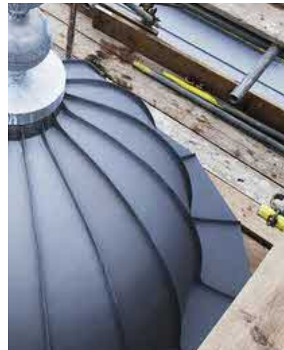
Metal Standing Seam Roof
