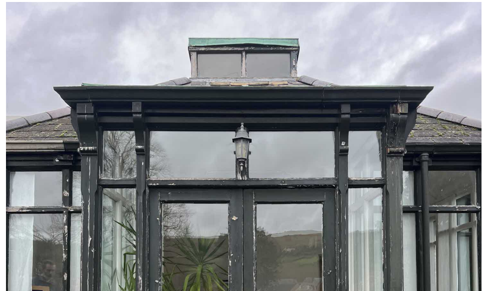
Fig 17. Original roof form replaced with a flat roof over porch
