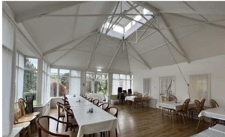
Fig 19. Existing conservatory currently used as for staff dining
