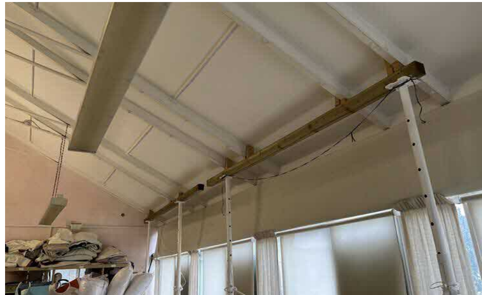
Fig 21. Acrow props supporting the existing structure
