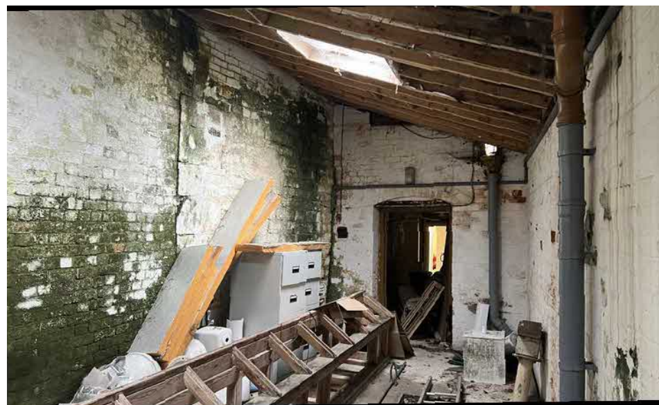
Fig 22. Room to rear where building meets neighbouring garage
