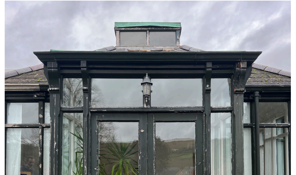
Fig 17. Original roof form replaced with a flat roof over porch
