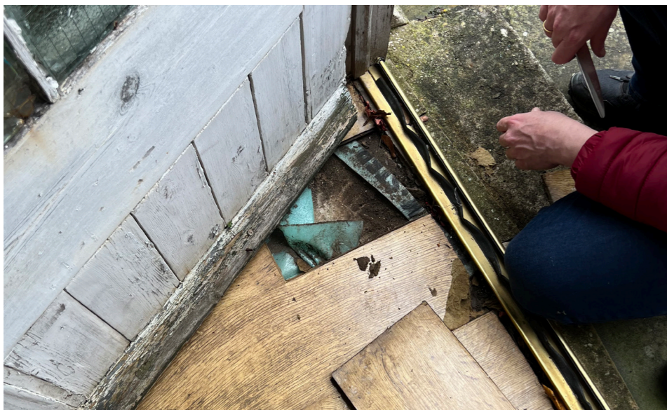
Fig 20. Concrete screed and laminate floor covering
