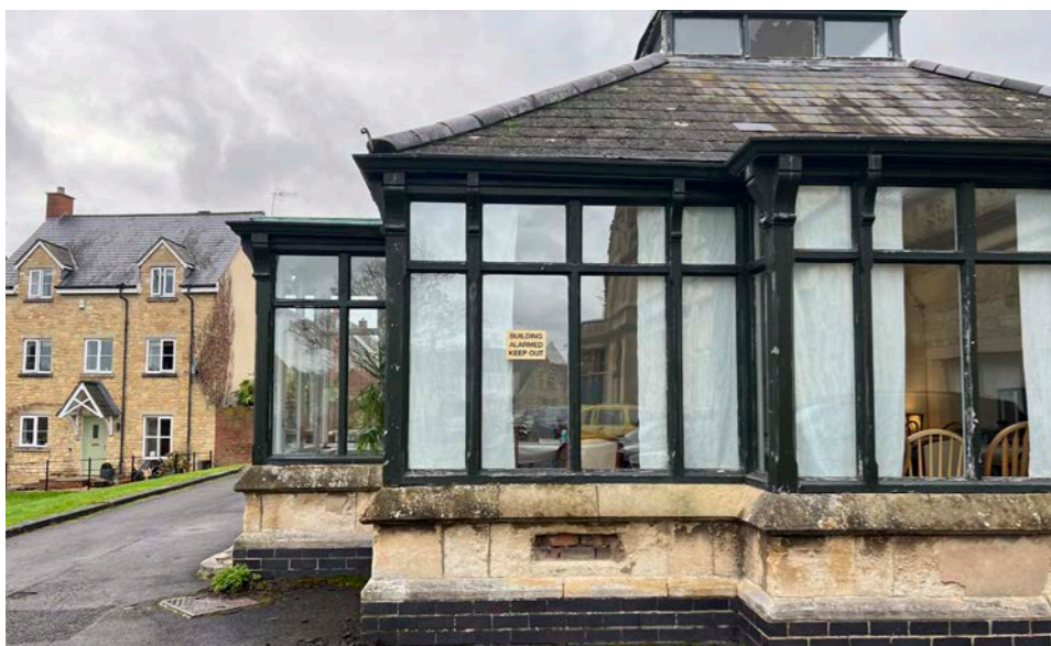
Fig 14. Existing conservatory east elevation
