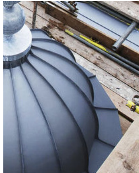
Metal Standing Seam Roof
