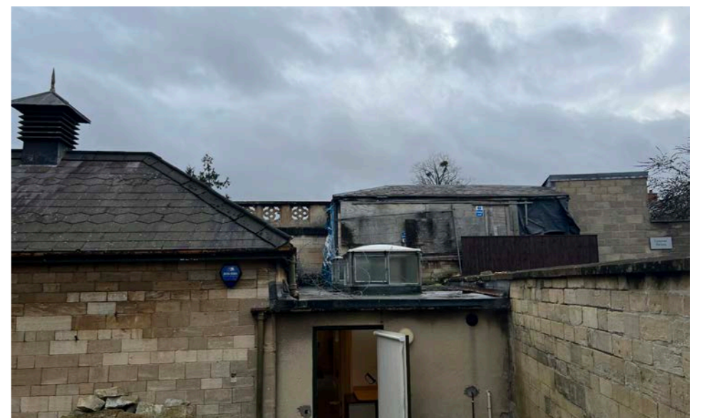
Fig 18. Rear of conservatory where building meets Ebley House
