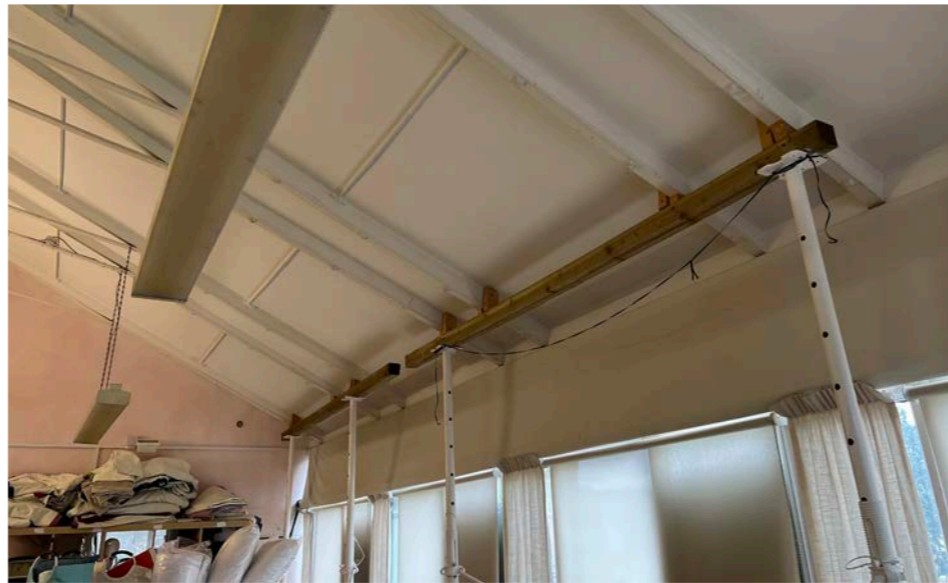
Fig 21. Acrow props supporting the existing structure
