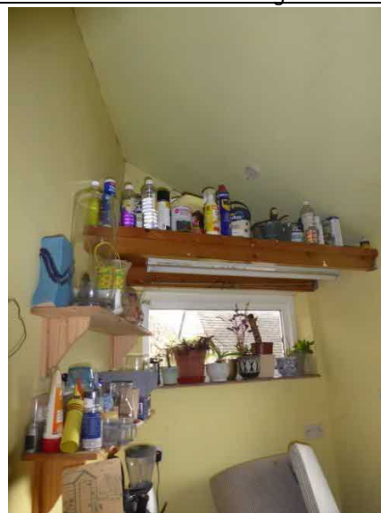
Inside of extension showing no loft space
