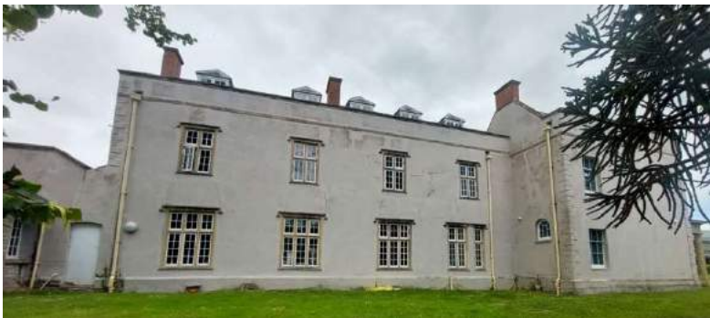
Fig. 5 South elevation of The Grange
