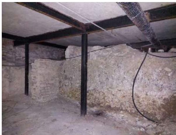
Fig. 41 Cellar beneath The Barn & Link buildings
