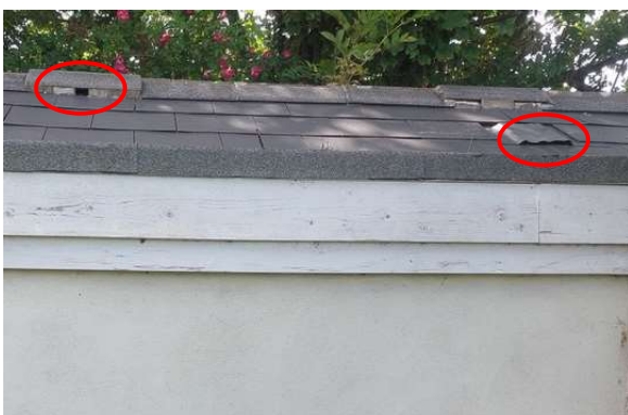
Figs. 82 and 83 Gap at ridge, bat access slate and bat tube on The Bat House
