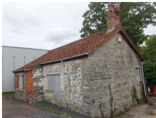
Fig. 45 South/west elevations of cottage
