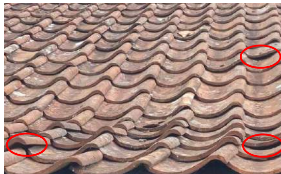
Figs. 74 and 75 Lifted and broken tiles on roof of Hodinott's Cottage
