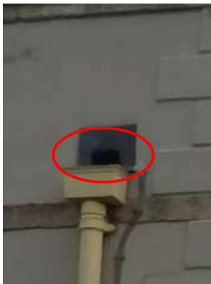
Figs 52 and 53 Gaps at top of drainpipes at The Grange
