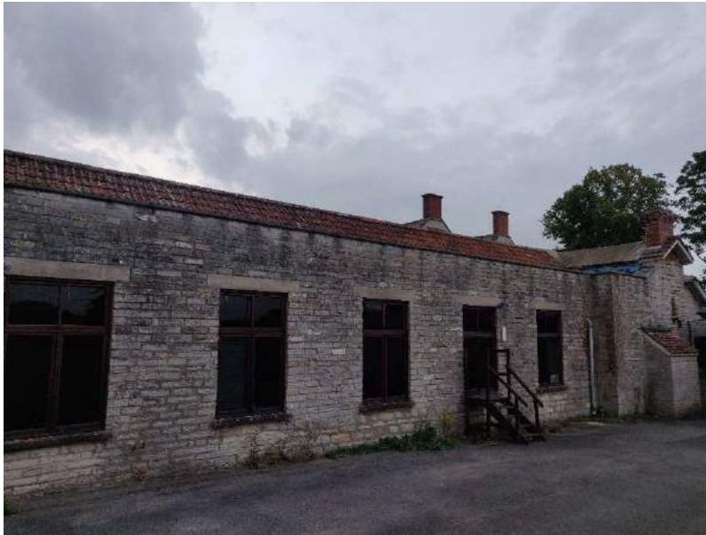
Figure 4 The west elevation of the Link Building
