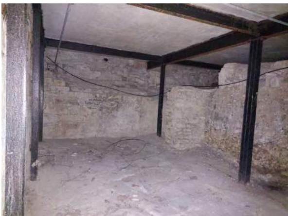
Fig. 42 Cellar beneath The Barn & Link buildings
