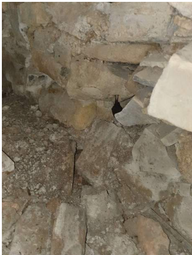
Fig.15 LHS bat in Back Cellar approx. 30cm from base of wall
