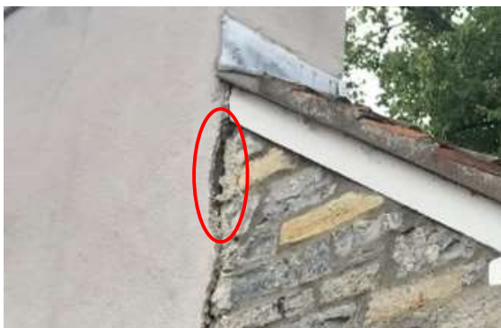
Figs. 54 and 55 Gaps to rear extension and at top of drainpipe
