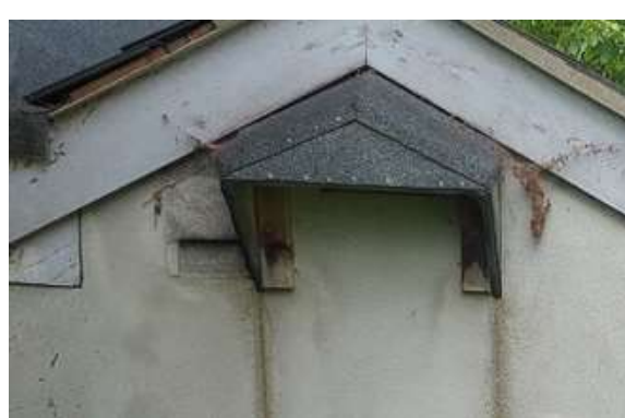
Figs. 82 and 83 Gap at ridge, bat access slate and bat tube on The Bat House
