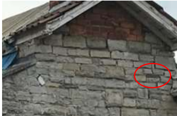
Figs. 64 & 65 Gaps in stonework of western elevation of The Link Building
