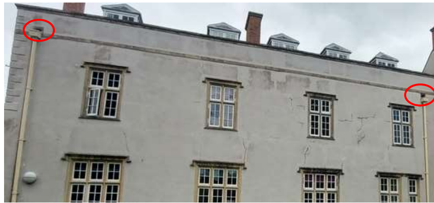
Figs 52 and 53 Gaps at top of drainpipes at The Grange
