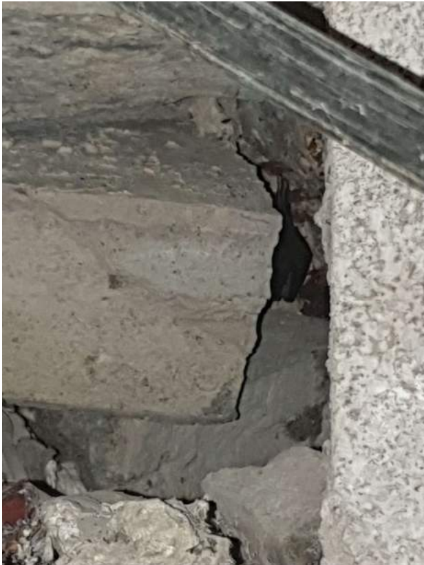
Fig.13 Lesser Horseshoe bat in hole in the wall of Back Cellar
