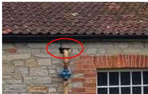
Figs. 54 and 55 Gaps to rear extension and at top of drainpipe
