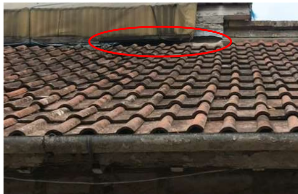
Figs. 62 & 63 Gaps in northern & southern sections of The Link Building roof
