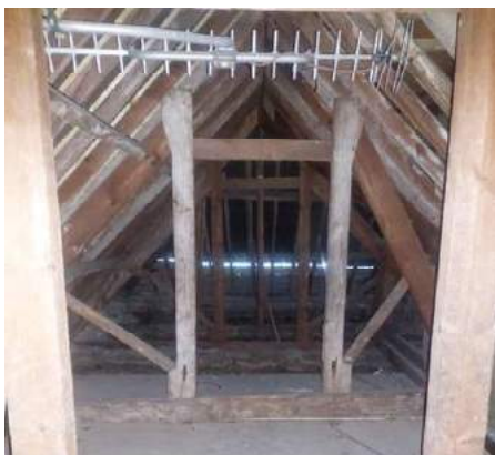
Figs 56 and 57 Gaps at the eaves of The Grange roof
