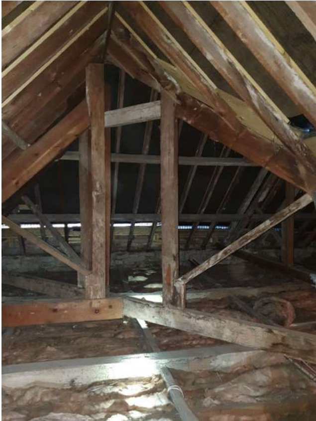
Fig.22 The Grange roof void
