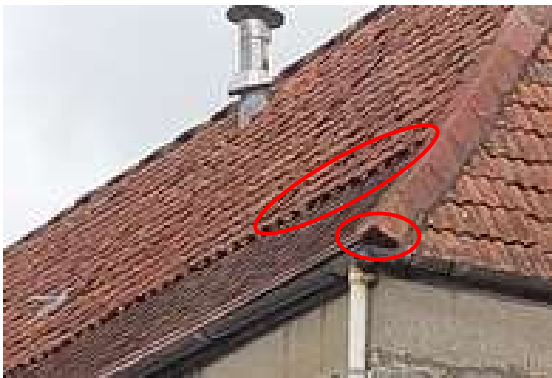
Figs. 70 and 71 Gaps under roof, hip and ridge tiles of The Barn roof
