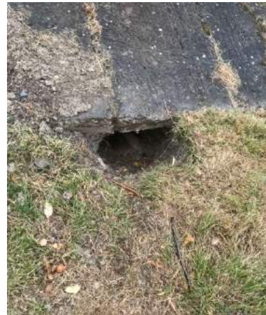
Fig. 3 Entrance hole B
