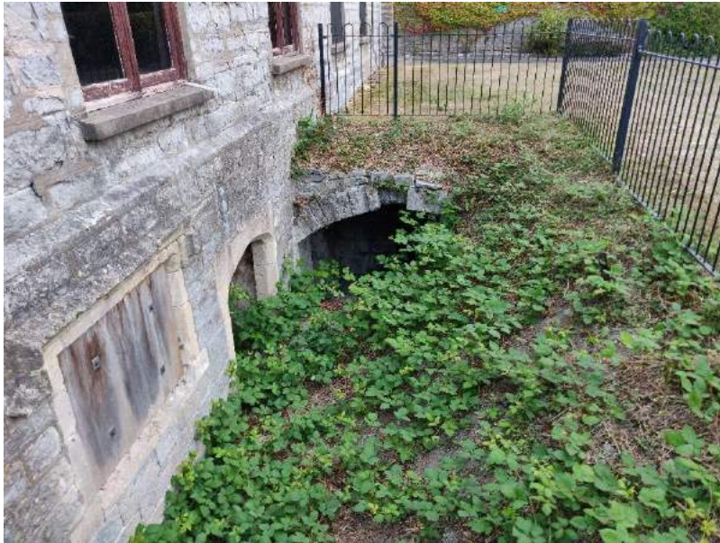
Figure 6 The entrance of the Tunnel
