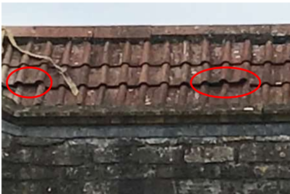
Figs. 62 & 63 Gaps in northern & southern sections of The Link Building roof
