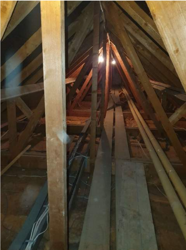
Fig.21 Link building northern roof void
