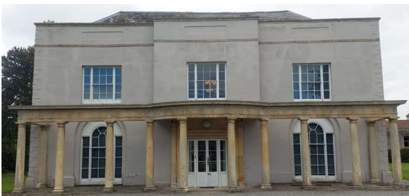
Fig. 4 East elevation of The Grange
