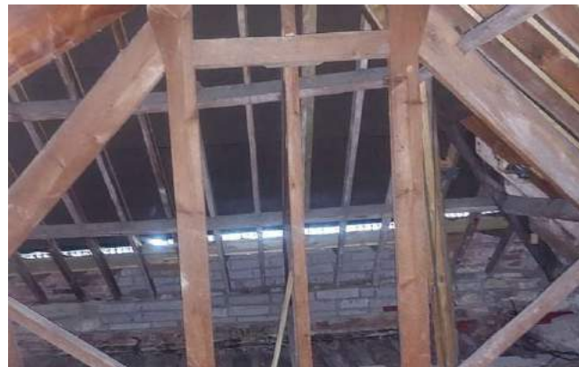
Figs 56 and 57 Gaps at the eaves of The Grange roof
