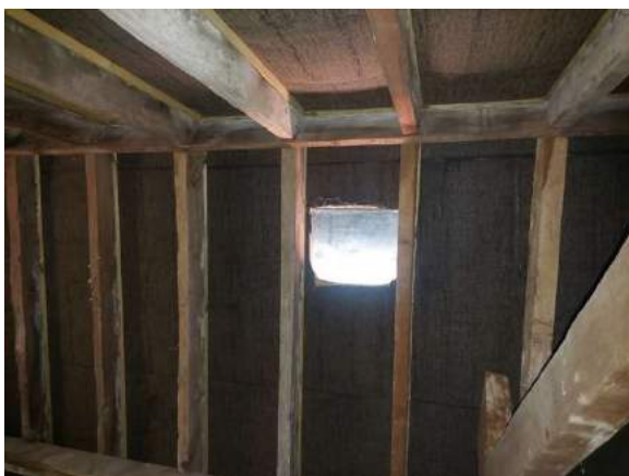
Fig. 58 Bat fly-in within The Grange roof
