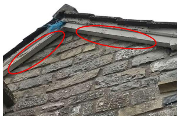
Figs. 66 & 67 Gaps under fascia and bargeboards of southern section of The Link Building
