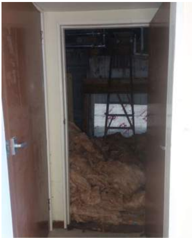
Fig. 16 Western roof void
