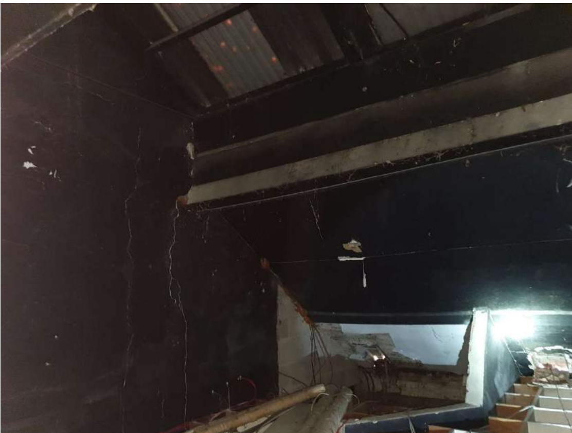
Fig.20 Link building southern roof void
