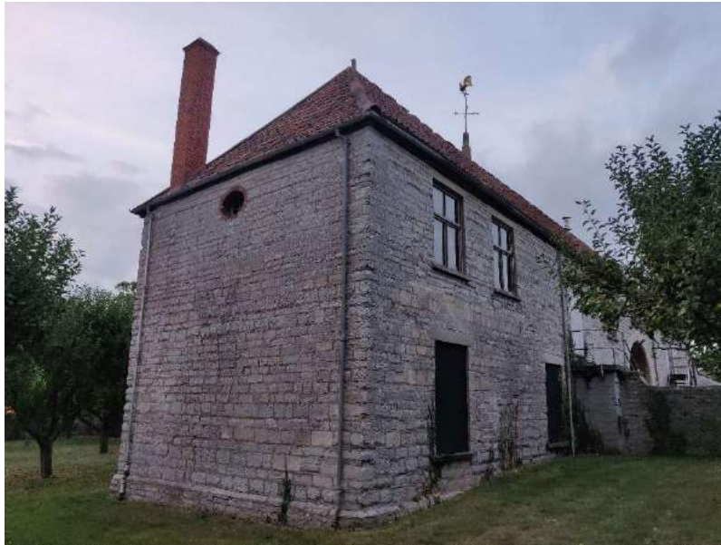
Figure 2 The north and west elevations of the Barn
