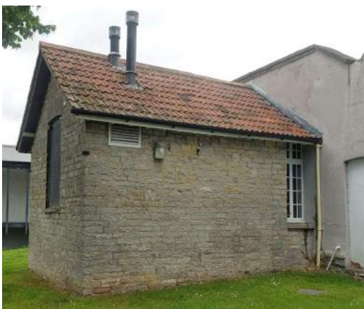
Fig. 6 Rear extension to The Grange
