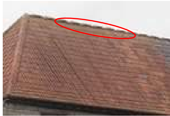
Figs. 70 and 71 Gaps under roof, hip and ridge tiles of The Barn roof
