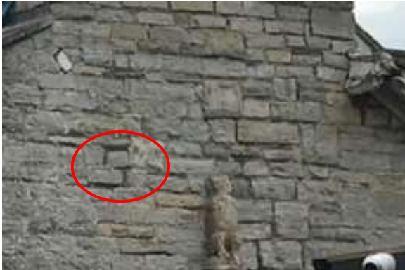
Figs. 64 & 65 Gaps in stonework of western elevation of The Link Building
