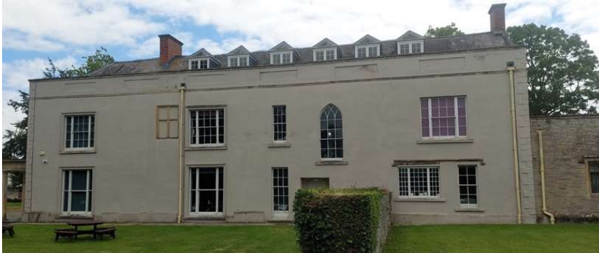
Fig. 3 North elevation of The Grange
