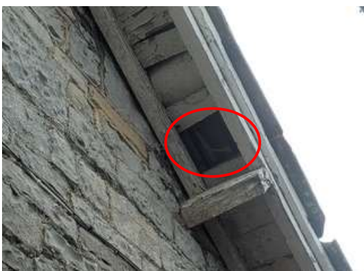
Figs. 66 & 67 Gaps under fascia and bargeboards of southern section of The Link Building
