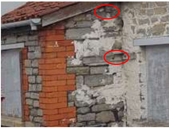
Figs. 76 and 77 Gaps in stonework and under soffits & fascia boards of Hodinott's Cottage
