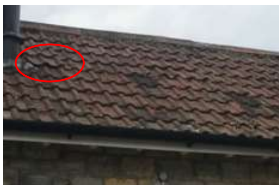
Figs 50 and 51 Gaps under tiles on rear extension roof
