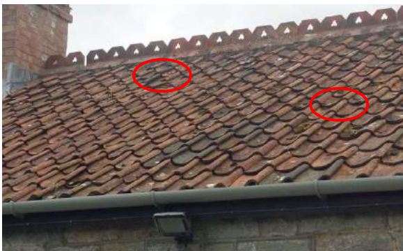
Figs. 74 and 75 Lifted and broken tiles on roof of Hodinott's Cottage
