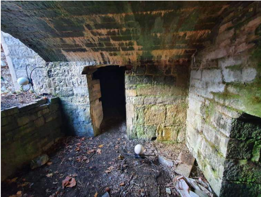
Fig. 6 Entrance Cellar showing entry to Back cellar (middle) & Tunnel (lower right)
