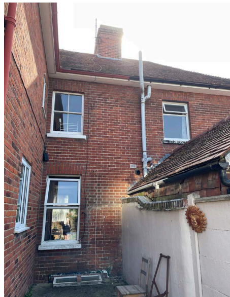
Site of proposed infill extension showing windows to be removed
