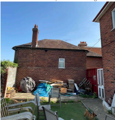
11a Vernon Place which forms Northern boundary
