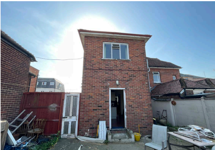
Rear elevation showing 11a Vernon Place to the left and boundary wall to the right
