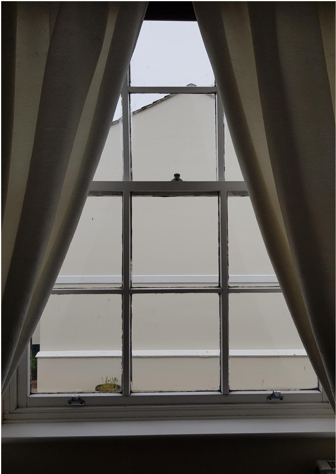
Internal View of Window and fittings
