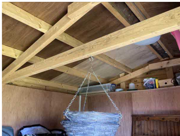
Interior stall (North end of building)
