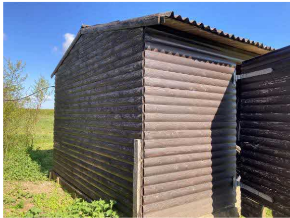
South facing gable end of the building
