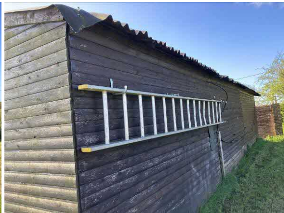
View of rear (west) of building
