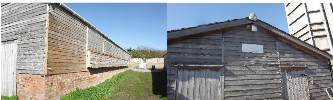
Figure 6 – Tongue and groove timber cladding (left), poultry house gable end and doors (right)
