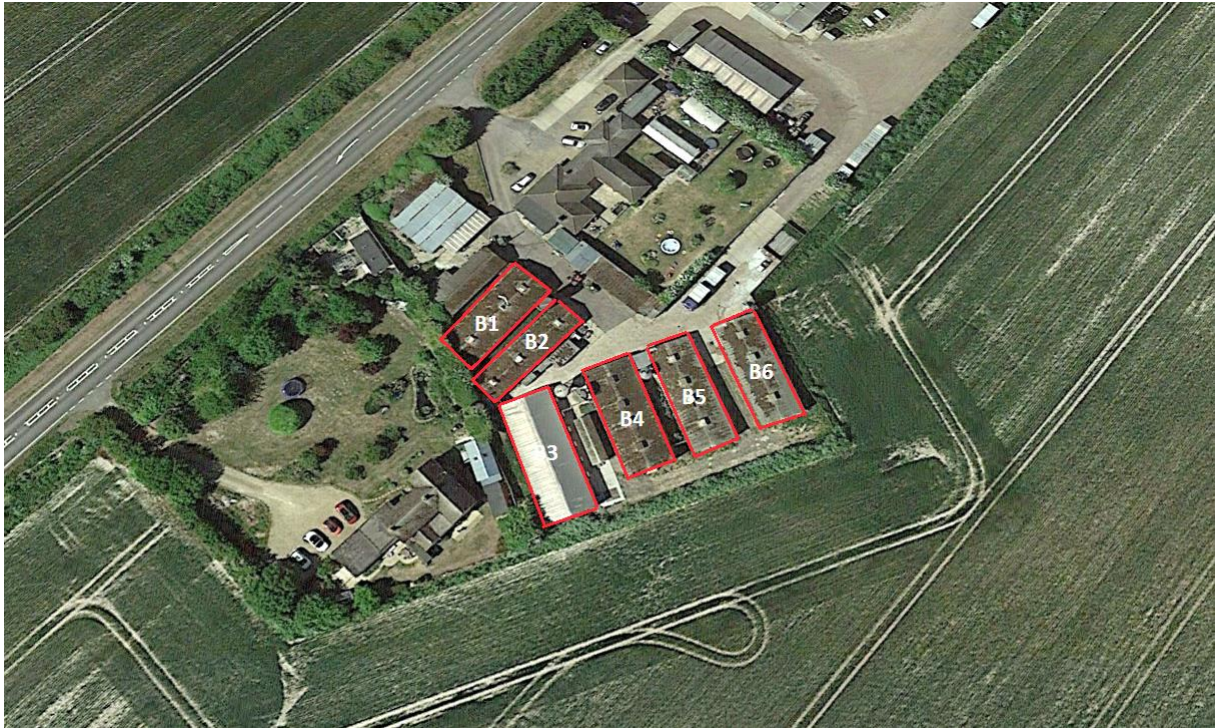
Figure 2 – Aerial View of Site and Buildings
