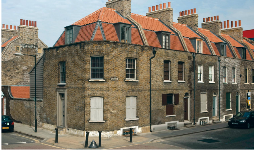
TURNER STREET IN THE SPITALFIELDS CONSERVATION AREA SHOWING TRADITIONAL LEAD DORMERS ON THE LISTED TERRACED HOUSES
