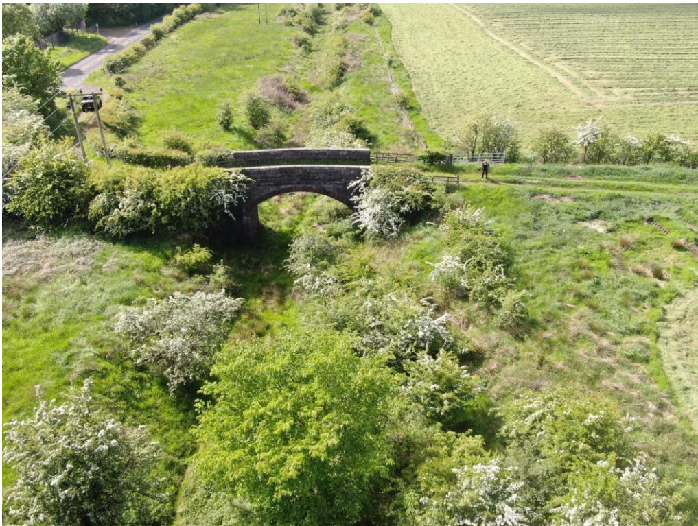
View of existing bridge (to be removed).
