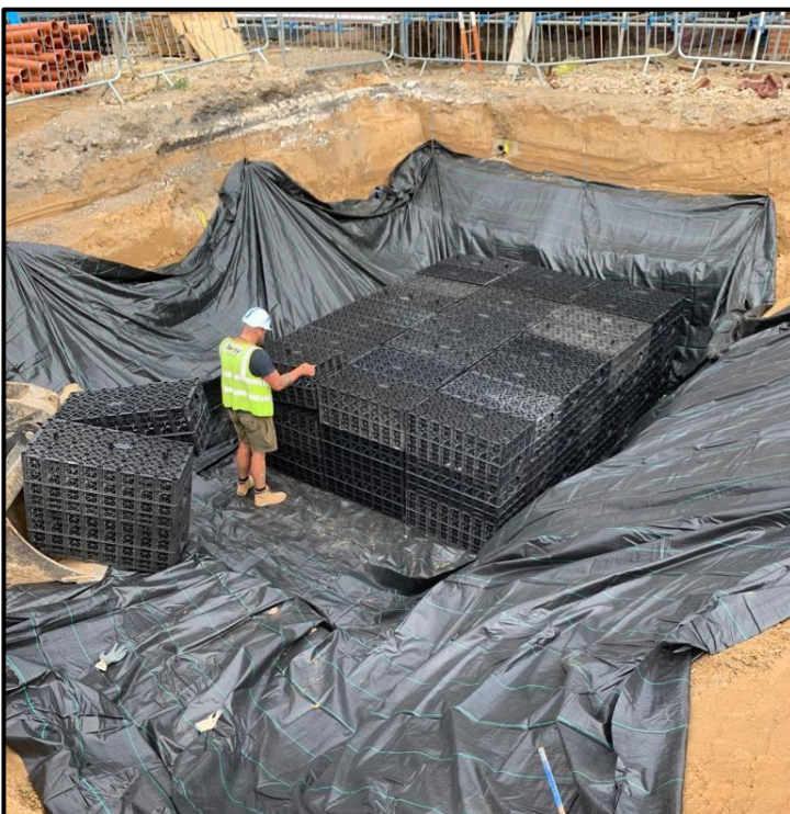
Figure 5 – Installation of attenuation crates (SA2)
