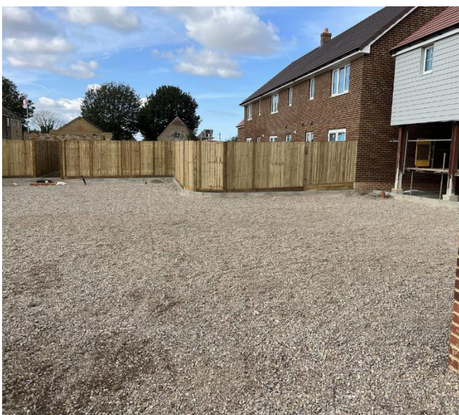
Figure 1 – 4-20mm stone sub-base in the courtyard to the rear of Plots 24 & 25.
