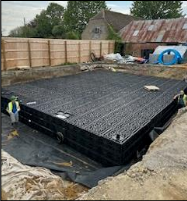
Figure 4 – Installation of attenuation crates (SA1)
