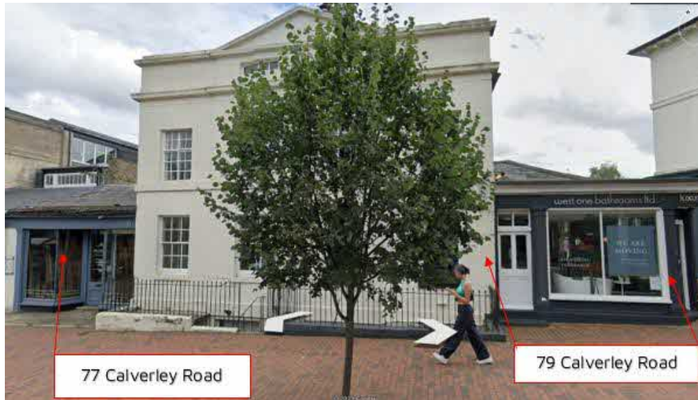
FIGURE 2.2: STREET VIEW OF SITE LOOKING NORTH FROM CALVERLEY ROAD
